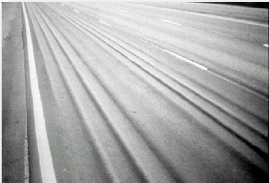
Figure 3.7. Surface depression in the wheel paths
