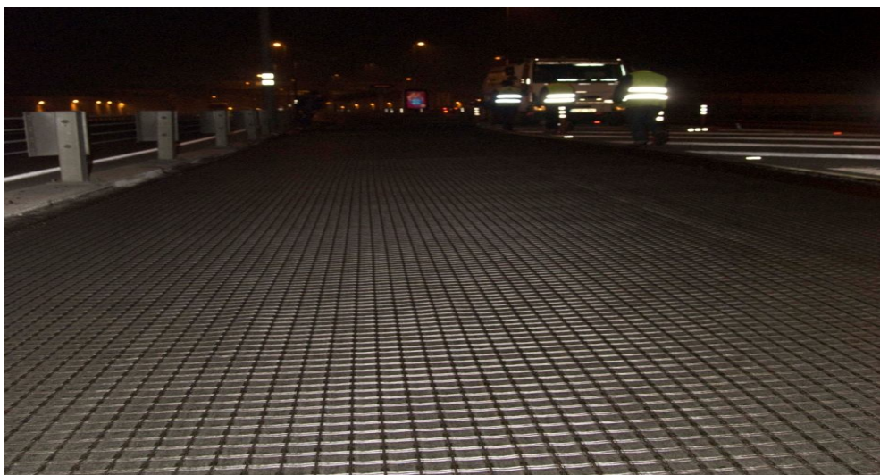
Figure 7.5. Geosynthetic application on METROBUS Line
