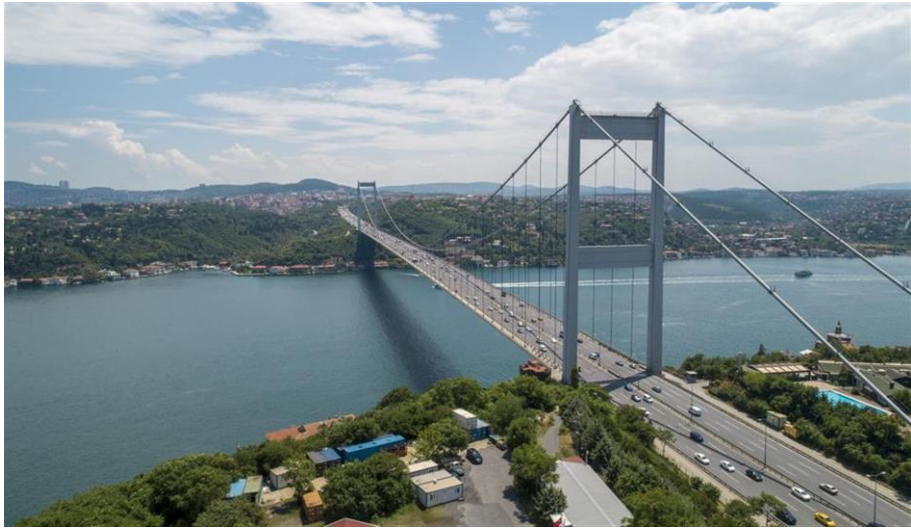
Figure 2.1. Location in aerial view of the FSM suspension bridge.
