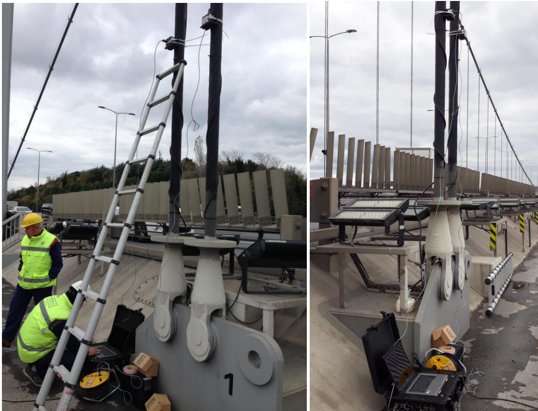
Figure 2.9. Temporary seismic network installation for longest hanger cable (strong motion accelerometer, transducer, power supply and laptop computer).
