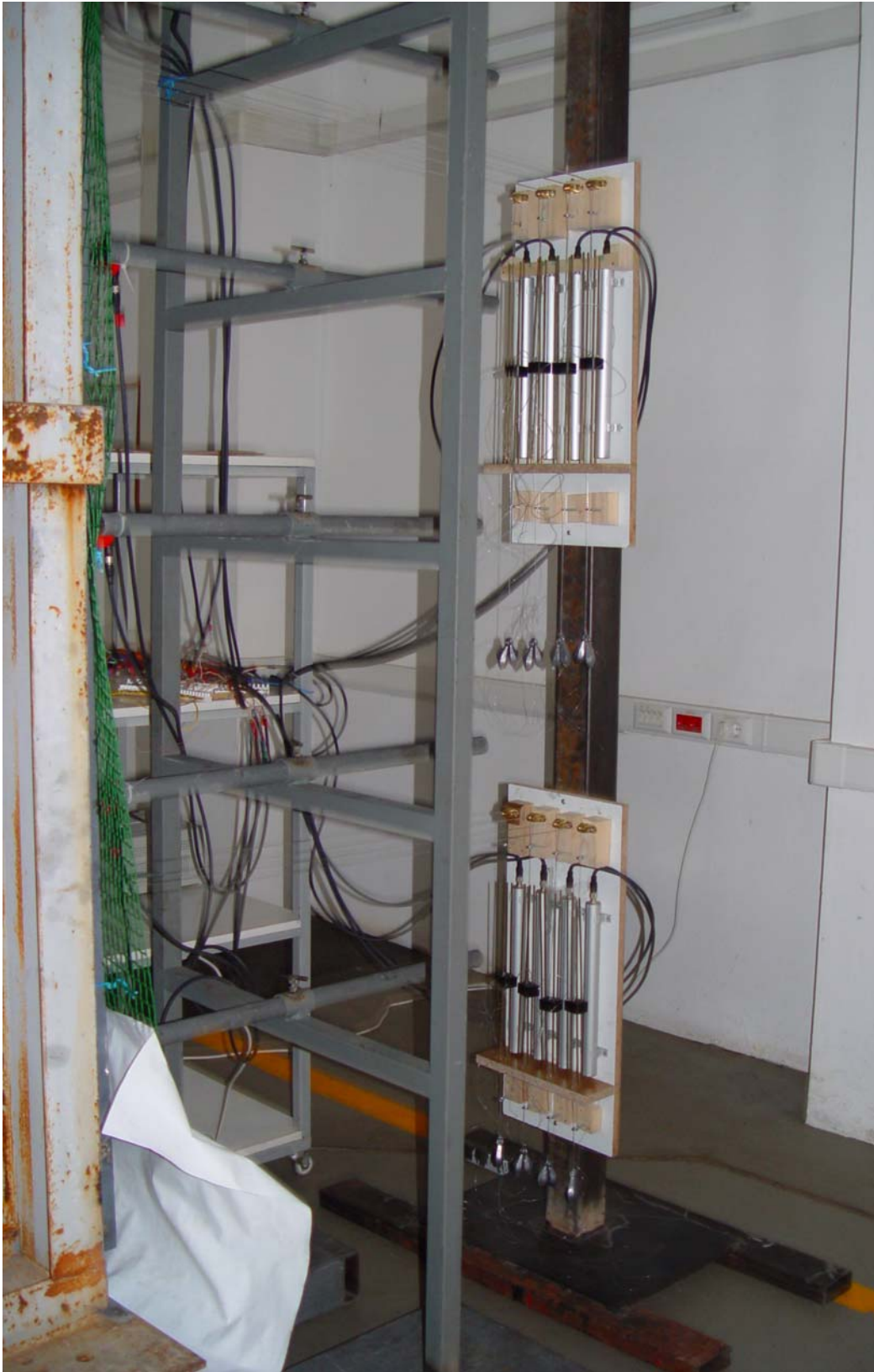
Figure 7.32. A general view of the posts
