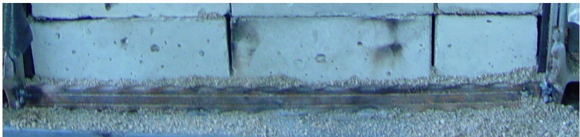
Figure 7.24. The wall's movement at the bottom was restricted by welding a piece of steel plate.
