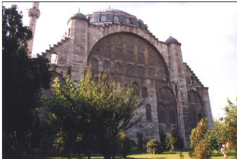
Figure 2.10. Exterior view of the Edirnekapi Mihrimah Sultan Mosque [22]
