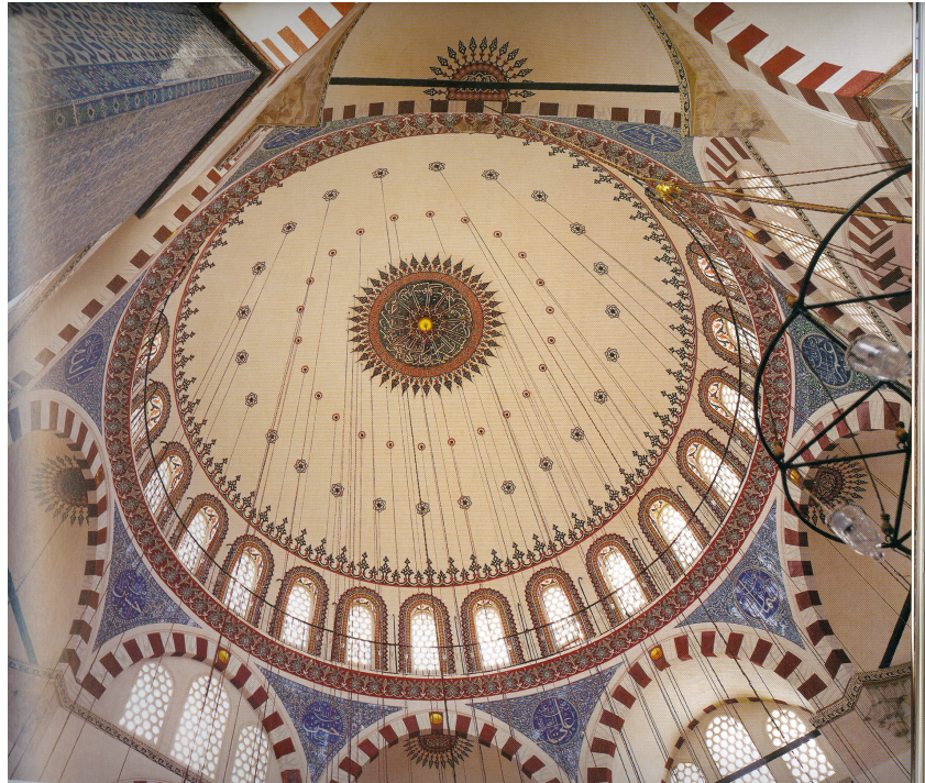
Figure 2.17. Interior view, looking up pendentives and dome [4]
