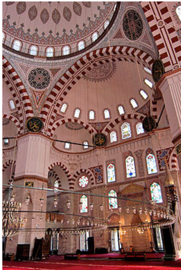
Figure 2.21. Interior view, looking up pendentives and dome [4]
