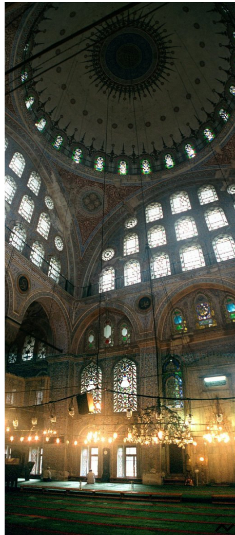
Figure 2.13. Interior view, looking up pendentives and dome [22]
