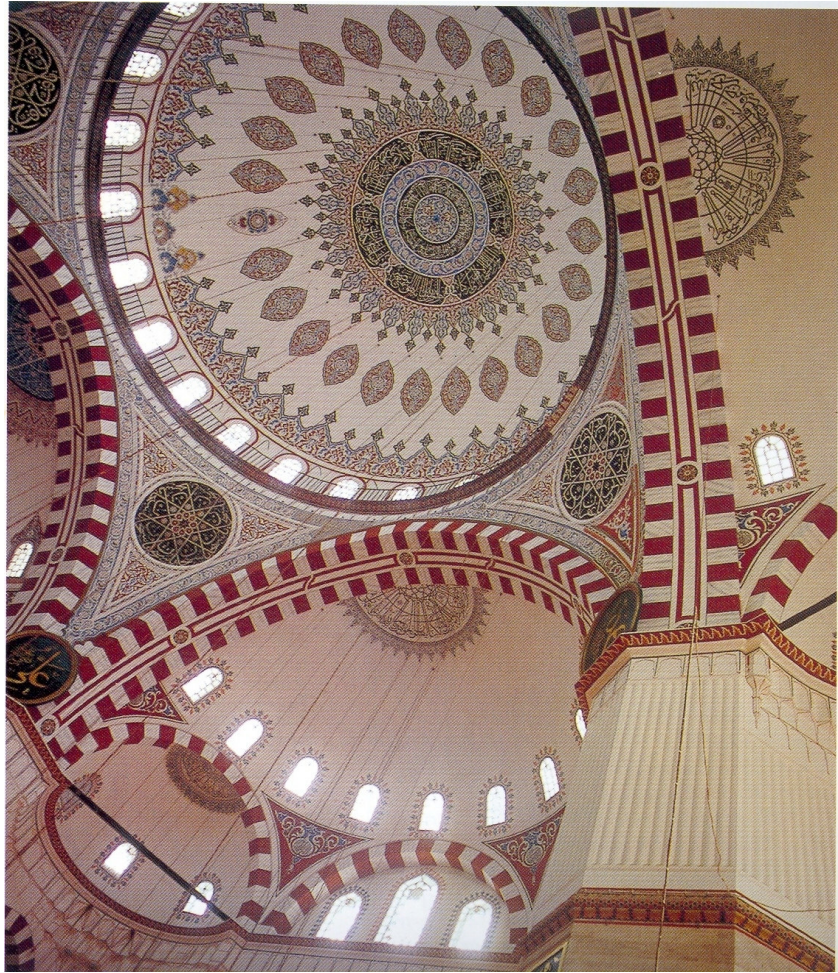
Figure 2.22. Interior view, looking up pendentives and dome [21]
