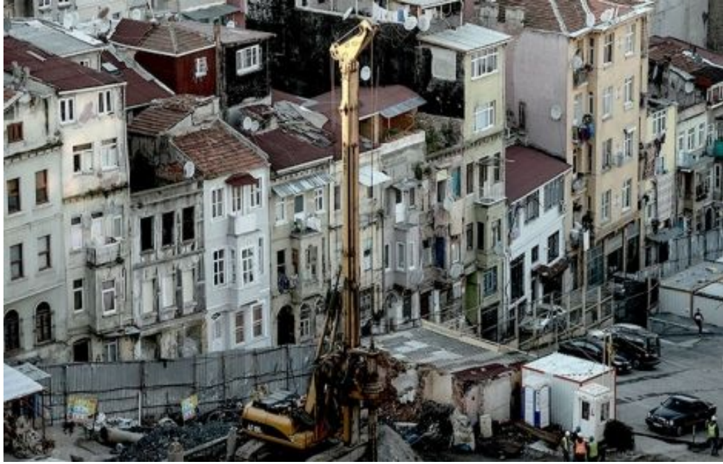
Figure 4. Demolitions in Tarlabası 35
