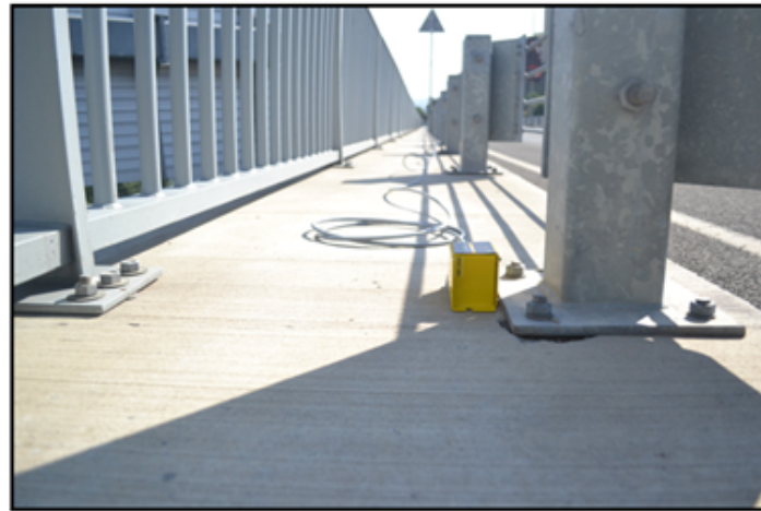
Figure 2.7. Short-term monitoring of the third column.
