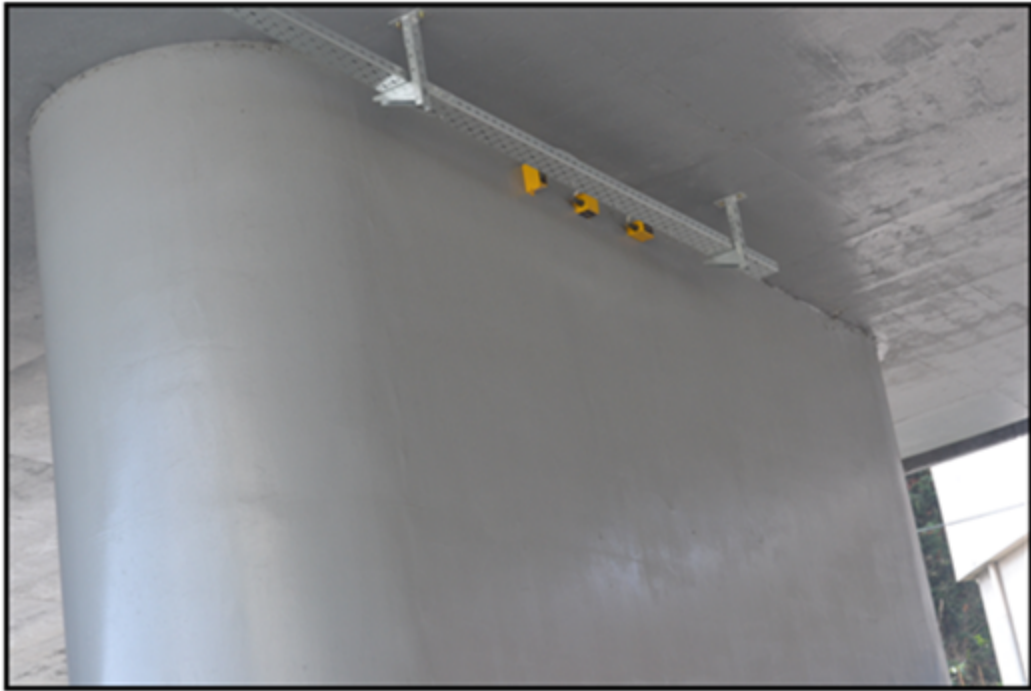
Figure 2.5. Sensors located on the first column.
