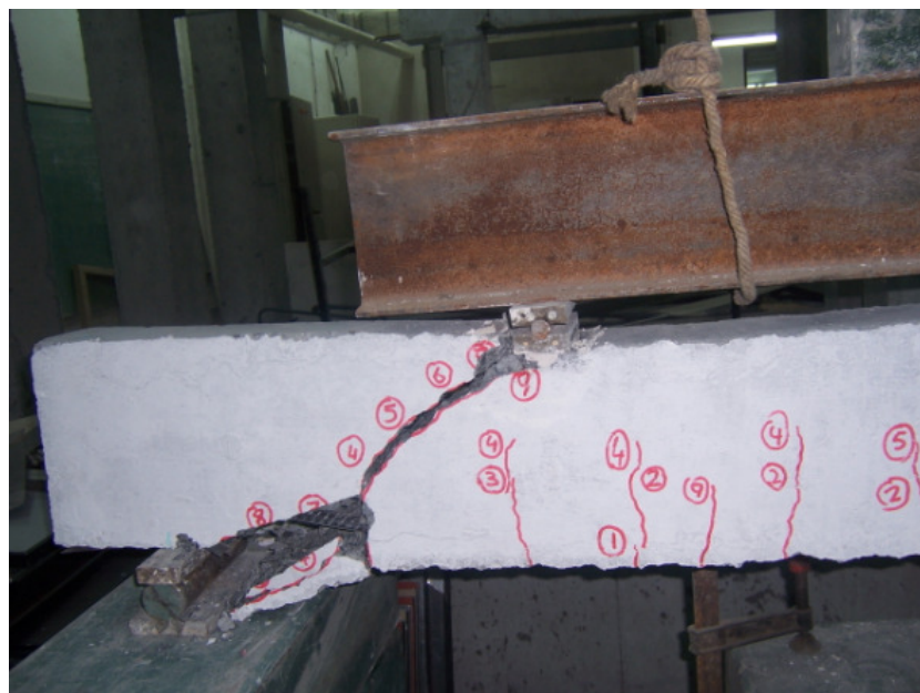
Figure 4.42. Damaged shape of the specimen BEAM-11
