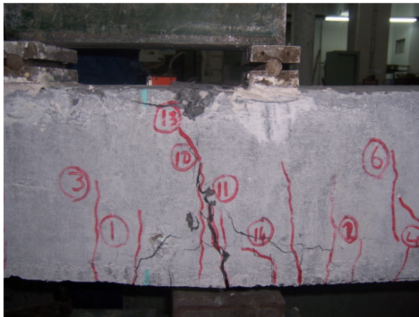
Figure 4.38. Damaged shape of the specimen BEAM-10
