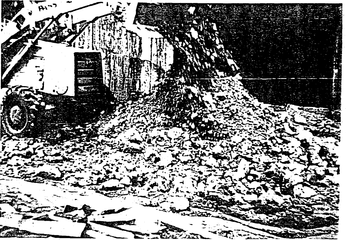
Photograph 1 Mixing the Soil with Lime
