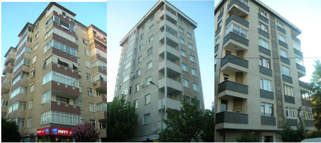
Fig. 1 1970s-80s Apartment Buildings (Bostancı- Maltepe, Istanbul).
