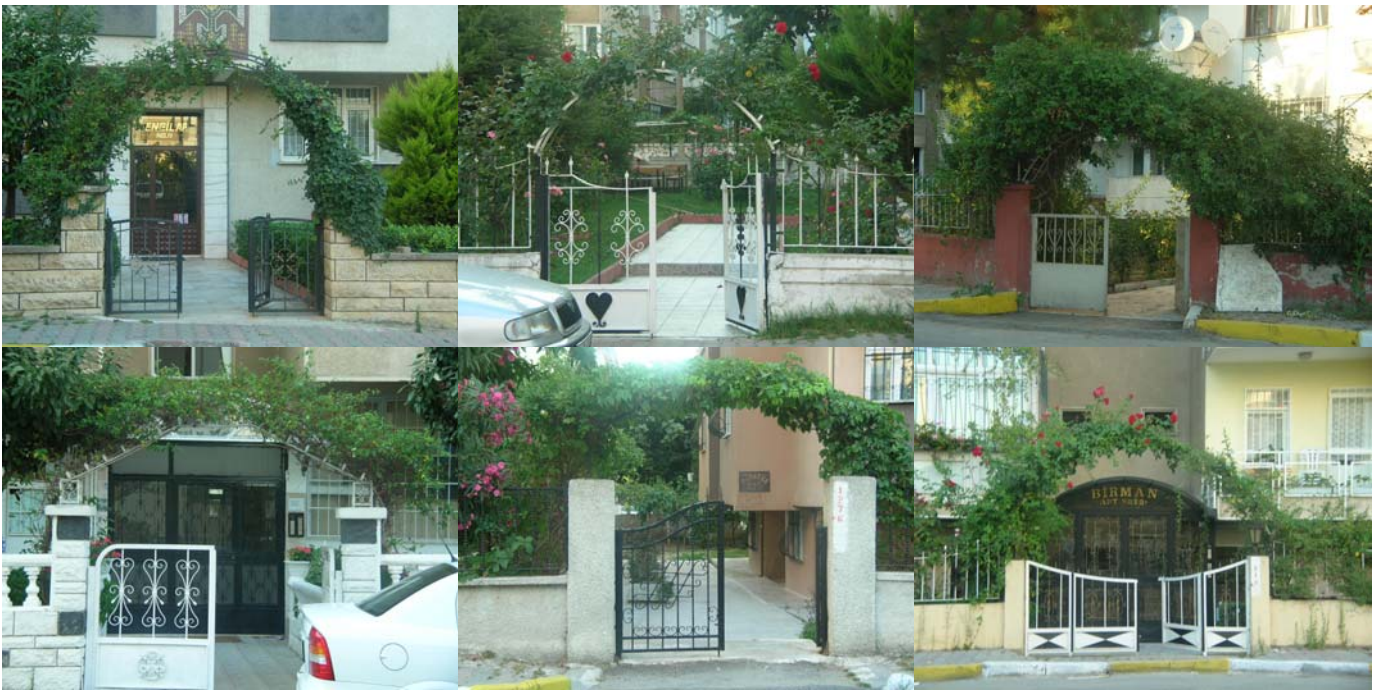
Fig. 11 Typical separate apartment building entrances.
