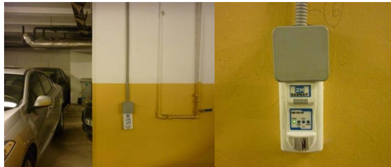
Figure 4.10. CO 2 detectors in the garage.
