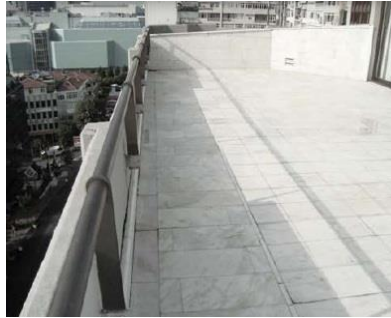
Figure 4.1. White tiles on the roof.
