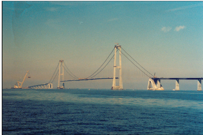
Figure 1.4. The Great Belt East Bridge in Denmark, center span 1624 meters (Virola, 2009)
