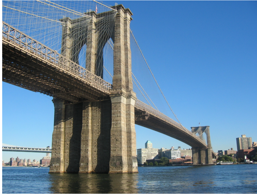
Figure 3.8. The Brooklyn Bridge in New York, U.S.A. (Commercial Office Space News, 2010)
