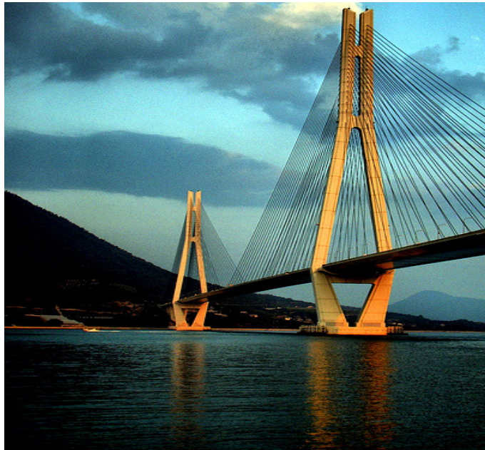
Figure 1.7. The Tataro Bridge in Japan center span of 890 meters (Virola, 2009)
