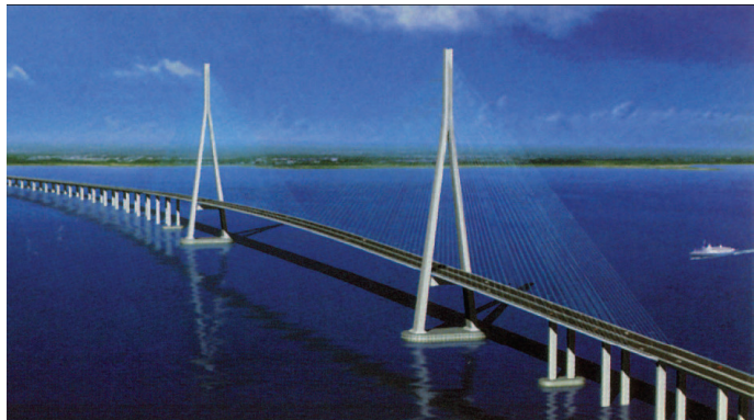
Figure 1.5. The Sutong Bridge in China, center span of 1088 meters (Virola, 2009)
