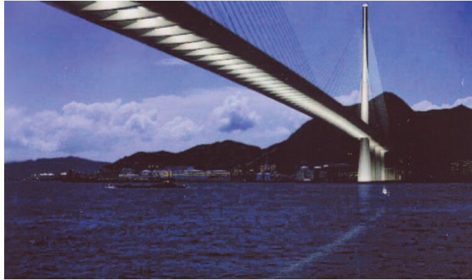
Figure 1.6. The Stonecutters Bridge in China, center span of 1018 meters (Virola, 2009)
