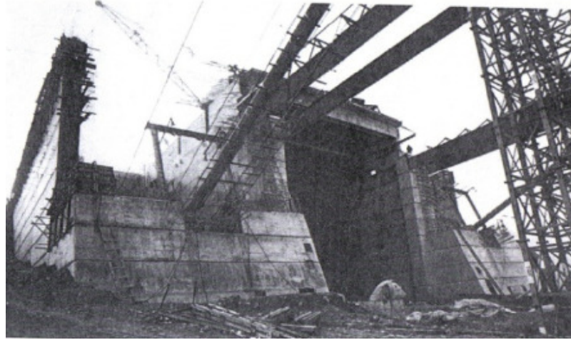
Figure 3.14. Anchorage block (Smith, 2009)
