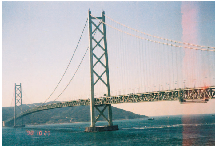
Figure 1.2. The Akashi-Kaikyo Bridge in Japan, center span 1991 meters (Virola, 2009)
