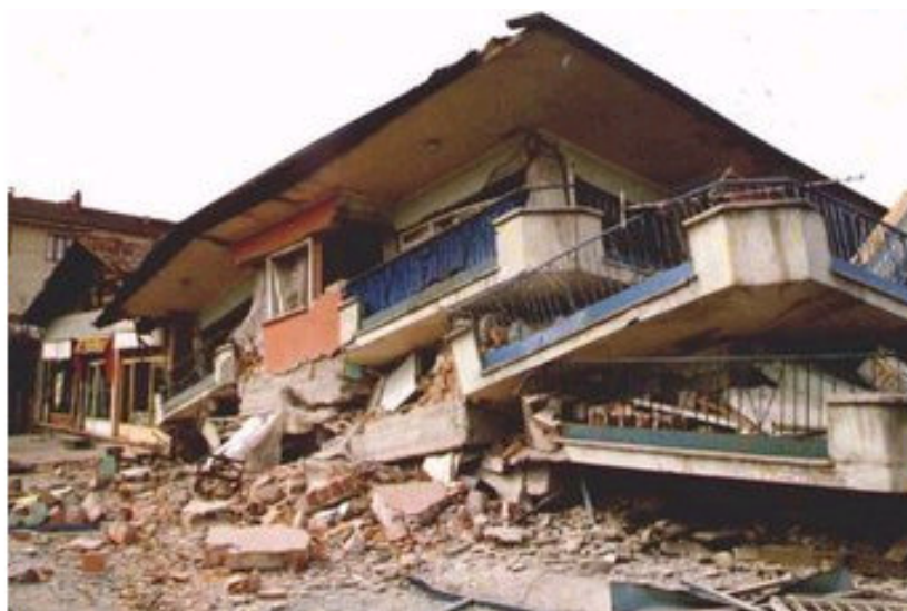
Figure 1.2. Collapse due to soft storey (1995 Dinar Earthquake)
