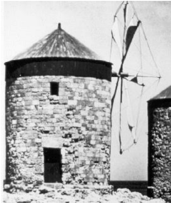
Figure 2.2. An Early European Horizontal Axis Windmill [24].
