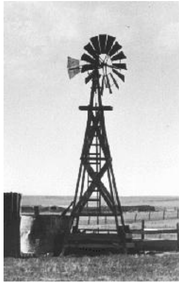
Figure 2.3. A Steel Blade Water Pumping Windmill [25].
