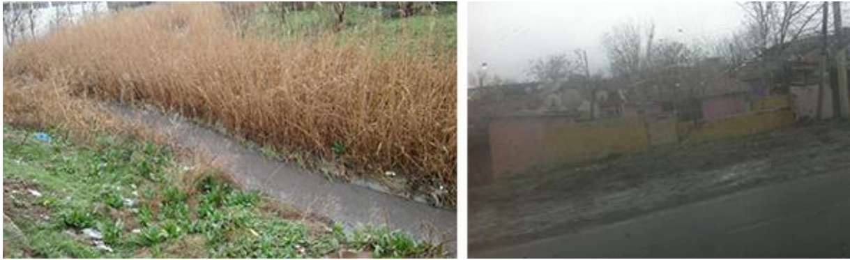
Figure 4.3. Çorlu Brook and shanty houses.
