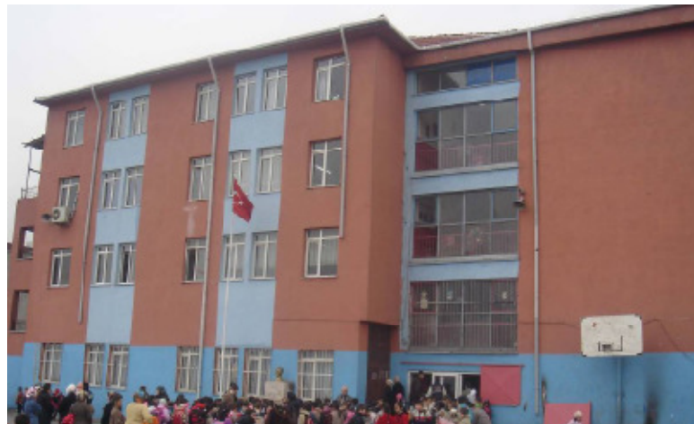
Figure 5.2. General view of Şehit Adem Yavuz Primary School building
