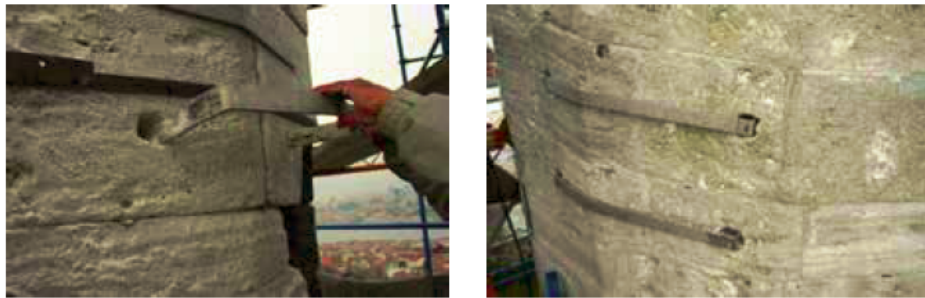
Figure 2.5. Application of stainless steel clamp
