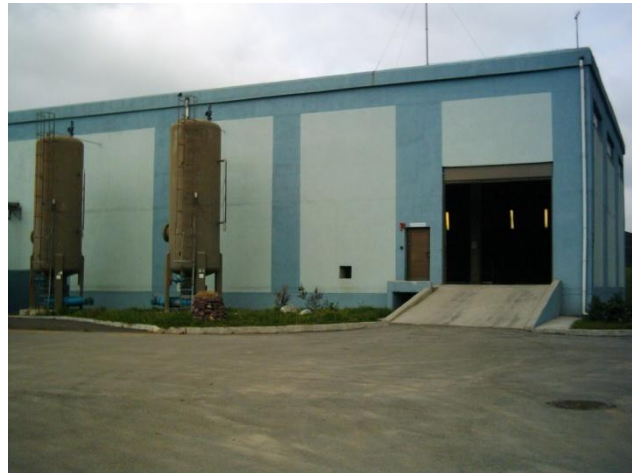
Figure 3.4. Pumping Station of Paşaköy WWTP
