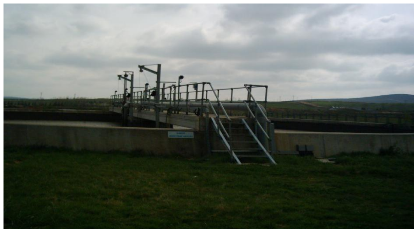
Figure 3.15. Sludge Storage Tank of Paşaköy WWTP
