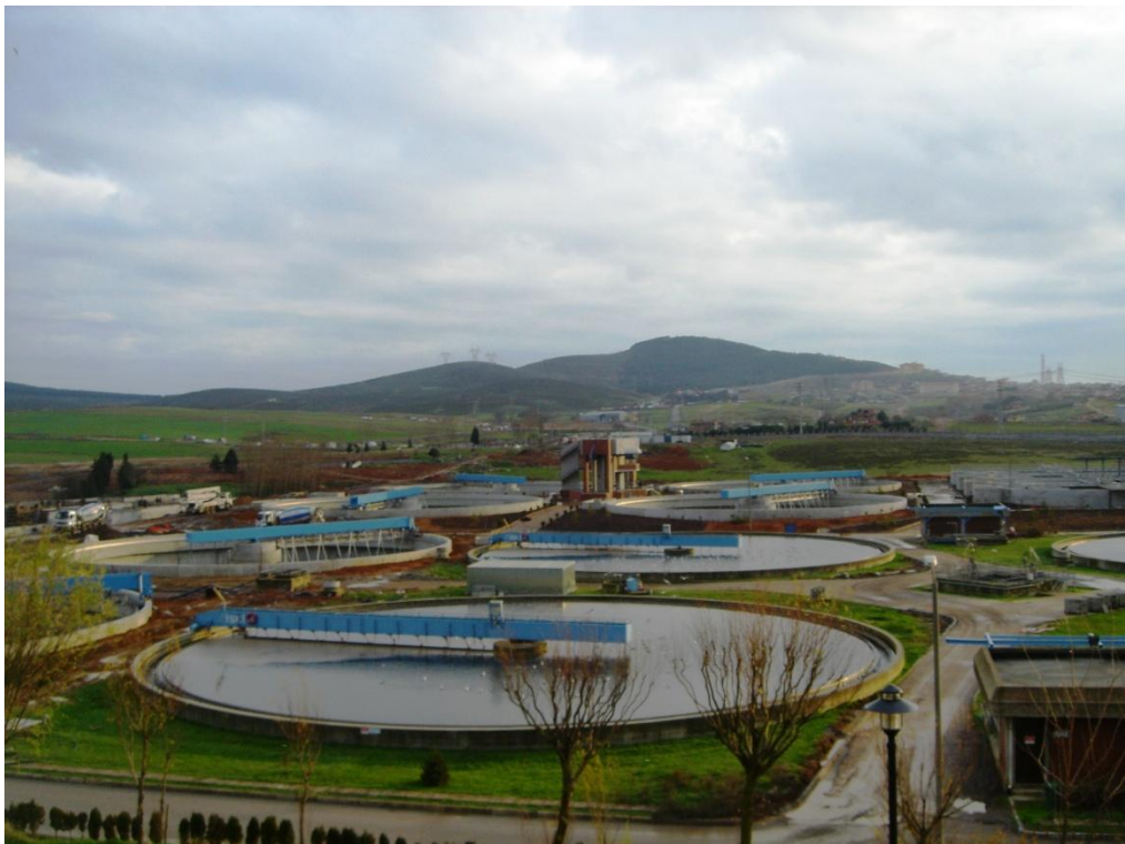
Figure 3.13. Final Clarifiers at Construction State
