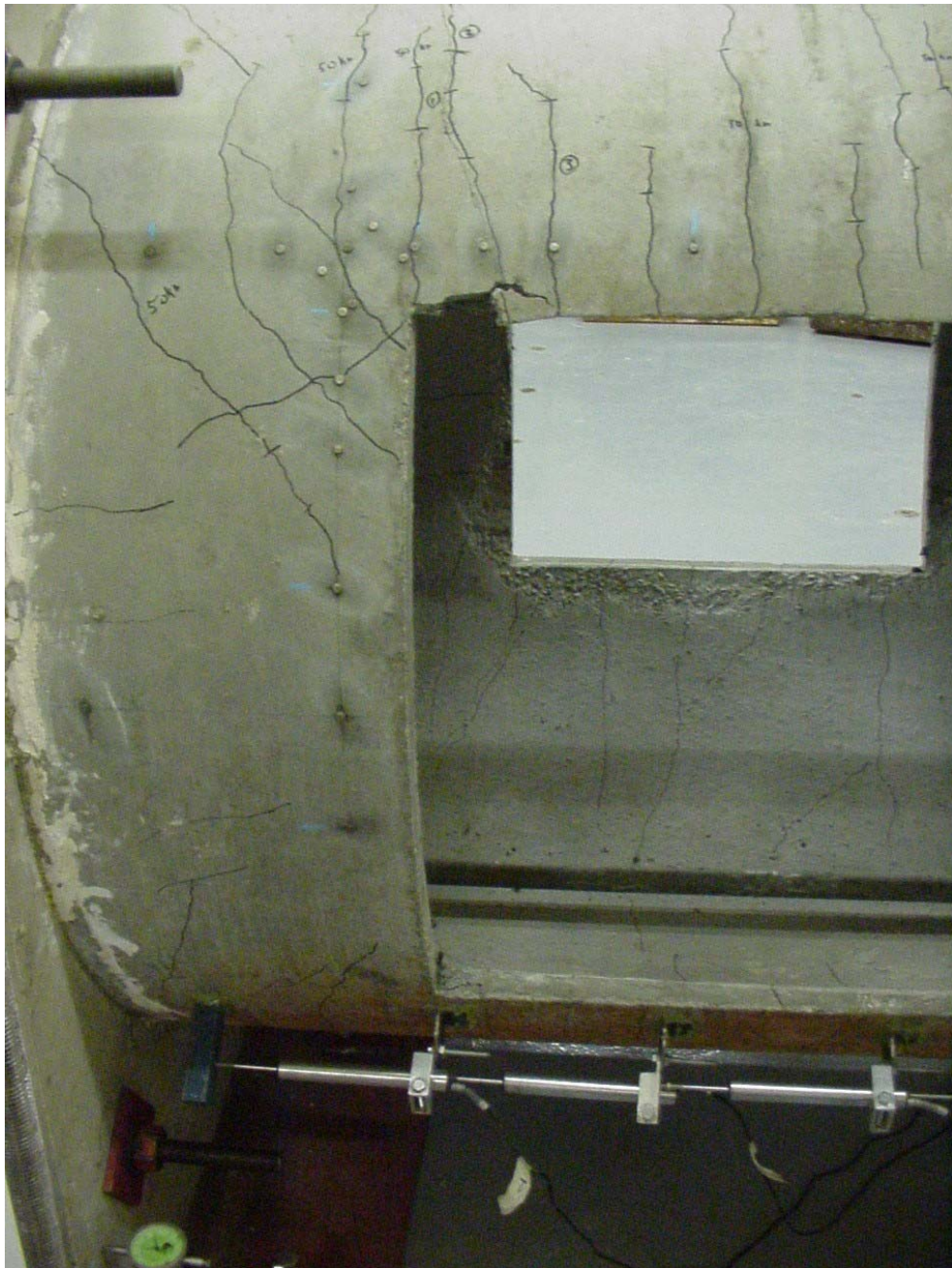
Figure 2.3. Bending Critical Case Damage [9].
