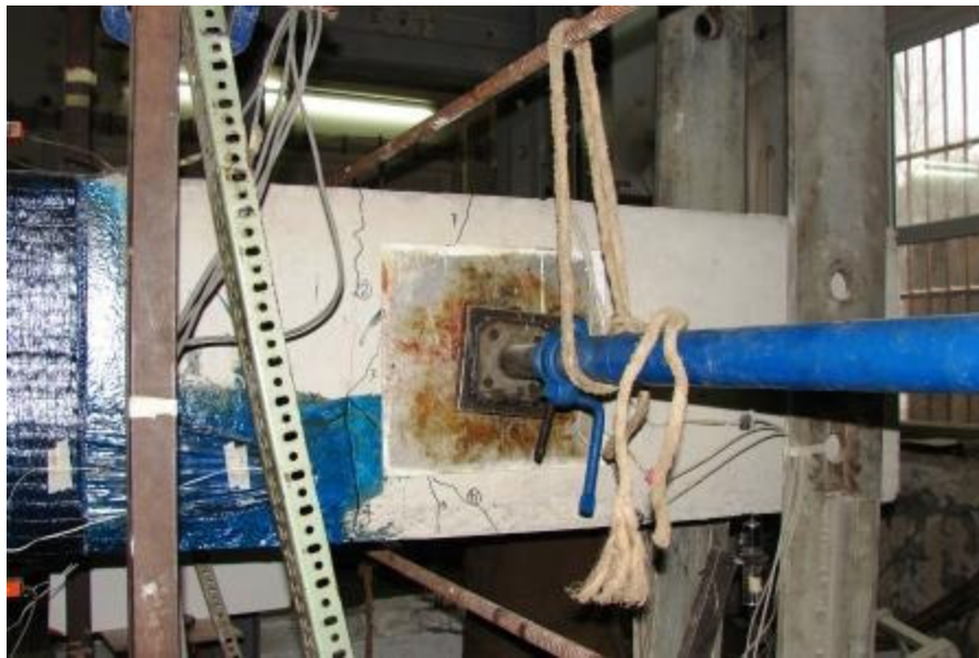
Figure 4.12. Crack pattern of US3-CS-FRP2 at the drift level of 1.40%
