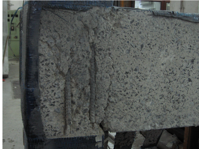
Figure 4.14. Image of the joint after the removal of FRP wraps
