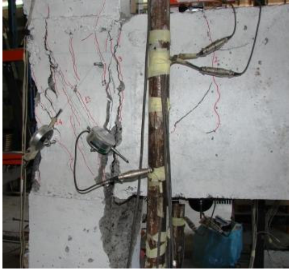
Figure 4.8. Failure pattern of US3-CS-Control
