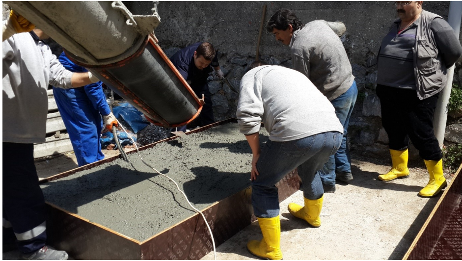
Figure 3.1. Ready mix concrete casting into molds.
