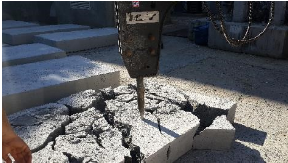
Figure 3.2. Concrete blocks prepared for transport to aggregate crushing site
