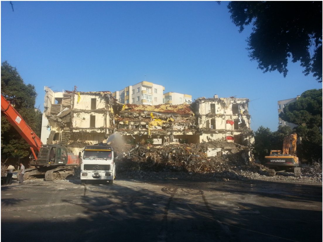
Figure 9. Demolishment began in Seyit Efendi High School
