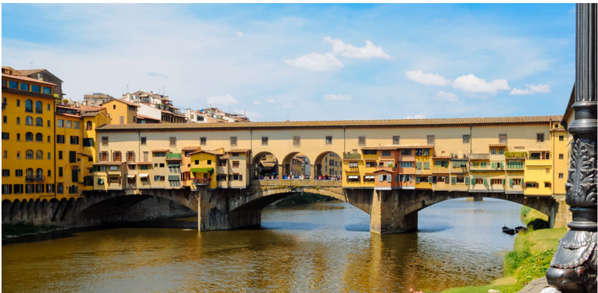
Figure 1.2. Ponte Vecchio Bridge [2]
