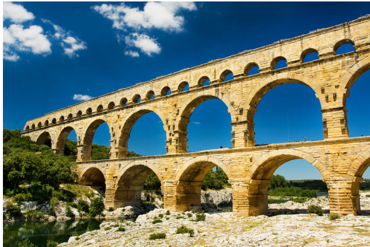
Figure 1.3. Pont du Gar Bridge [3]
