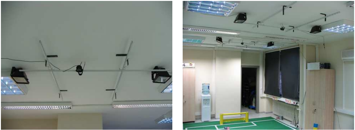
(a) Ceiling installation
