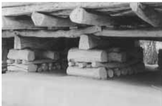
Figure 2.2. Use of Timber as Base Isolator (Hussain, 2014).
