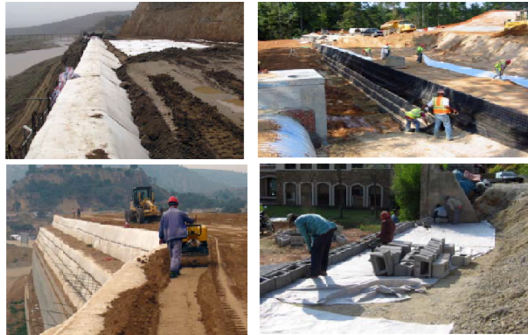
Figure 2.3. Scenes from Construction Steps of MSEWs (Tencate, 2012).
