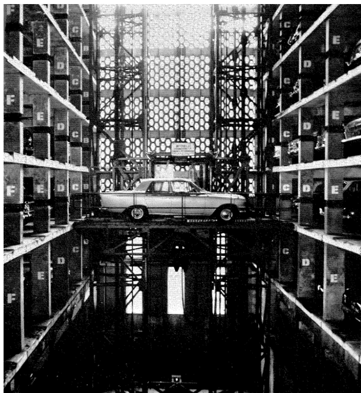
Figure 2.15. An early example of concrete AVPS in the 1970s (Dobson, 1974)
