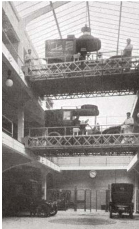
Figure 1.1 The first car stacker: Garage Rue de Ponthieu, 1905, Paris (Parking-net, 2020)
