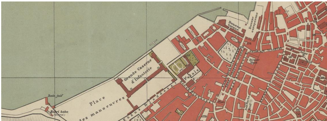
Fig. 56 Newly constructed area on the left side of the Ottoman custom
