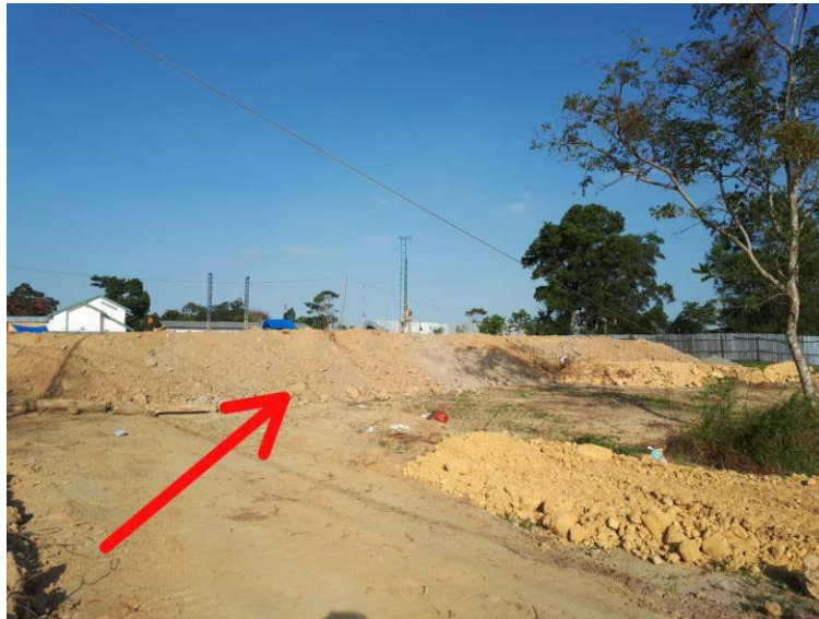
Figure 1. Construction site with clay as embankment material to raise ground level
