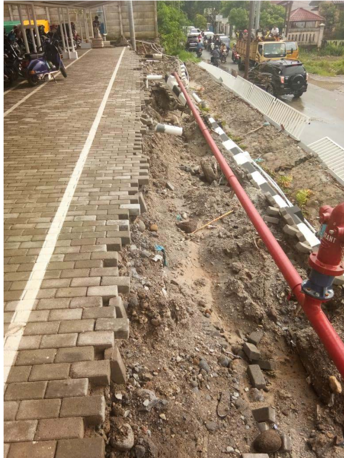
Figure 4. Example of fill material failure
