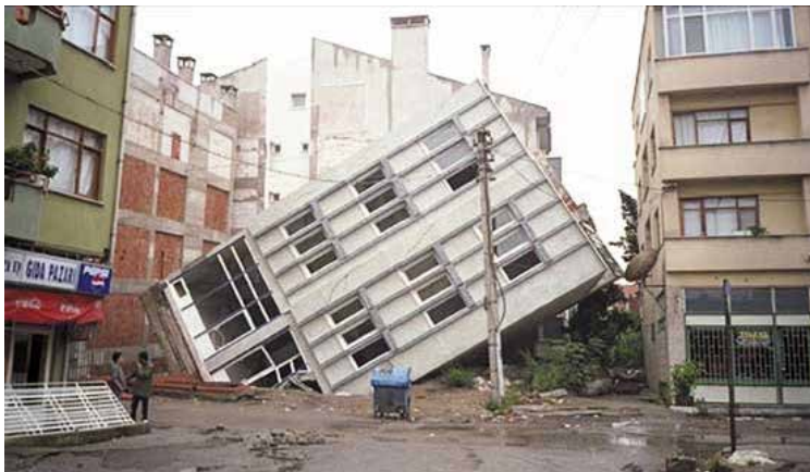
Fig. 1. Partially overturned building in Adapazari, Turkey during the 1999 Kocaeli (Izmit) earthquake because of liquefied and weakened soil beneath
