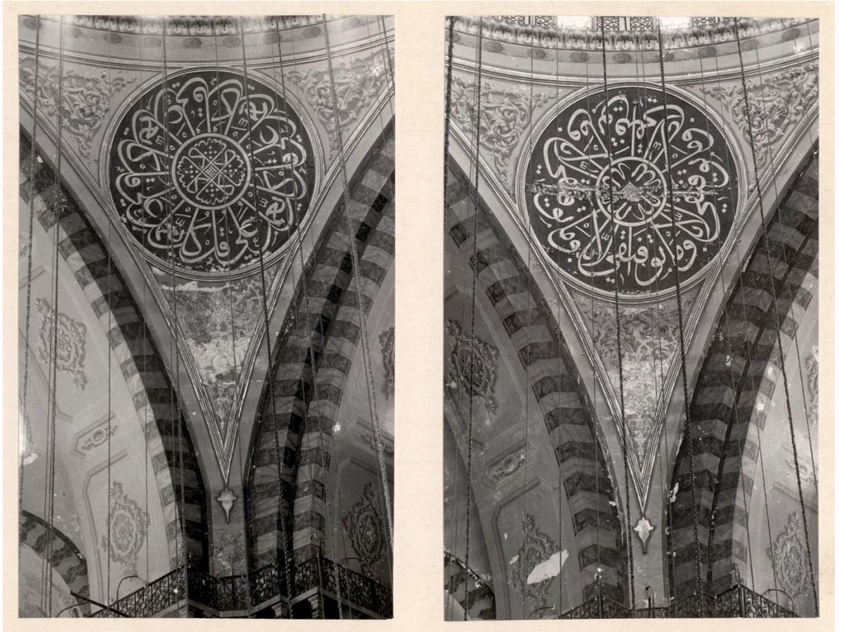
Figure 56. Photographs from the restoration of the Süleymaniye Complex (3)
