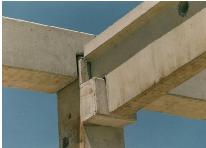
Figure 1.2. Roof girder-column connection [4].
