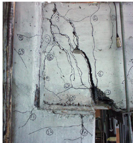
Figure 2.4. Damage in composite connection specimen at 3.5% storey drift level.
