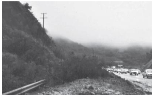
Figure 2.3. Flow slide on Highway 24 (Duncan, 2005).
