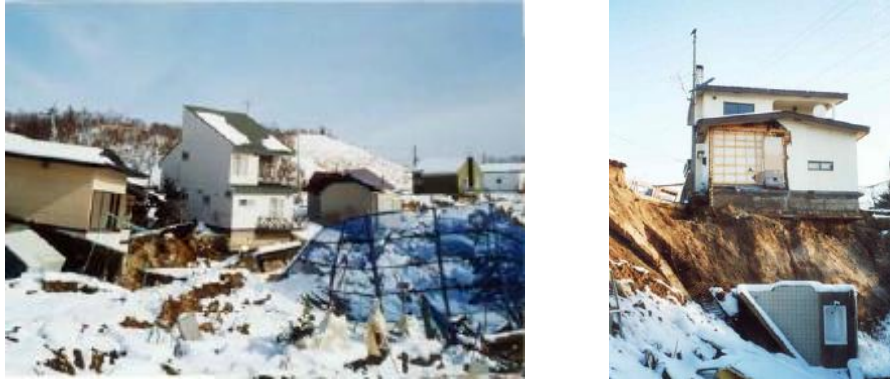
Figure 5.6. The residential area located on the failed embankment (Towhata, 2008).
