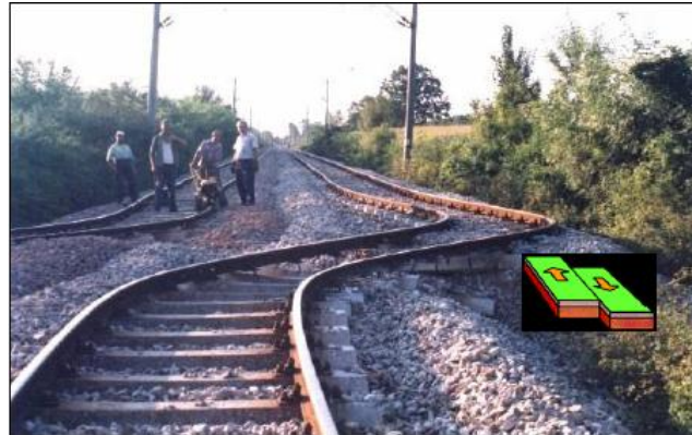
Figure 2.7. Fault displacement after the 1999 Kocaeli Earthquake.
