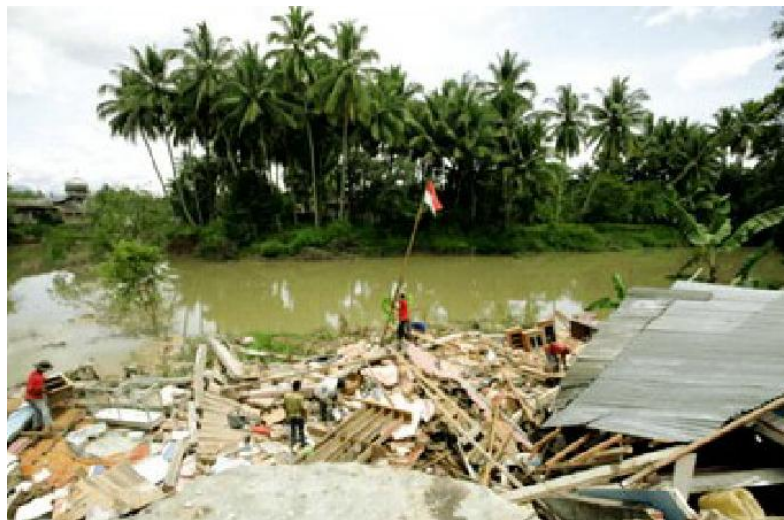
Figure 5.9. Collapsed neighbourhood of Sumatra located on the failed embankment (Japan Society of Civil Engineering Reports, 1998).
