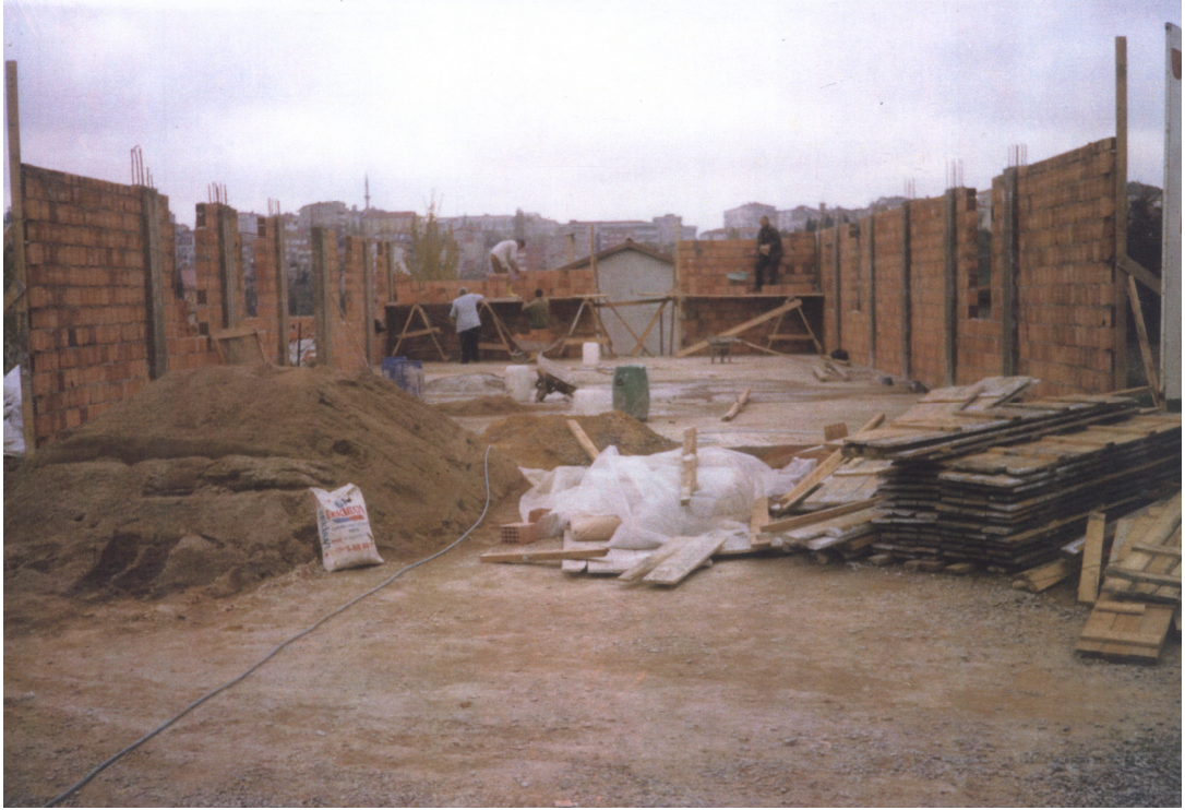
Fig. 5. Construction of Cemevi
