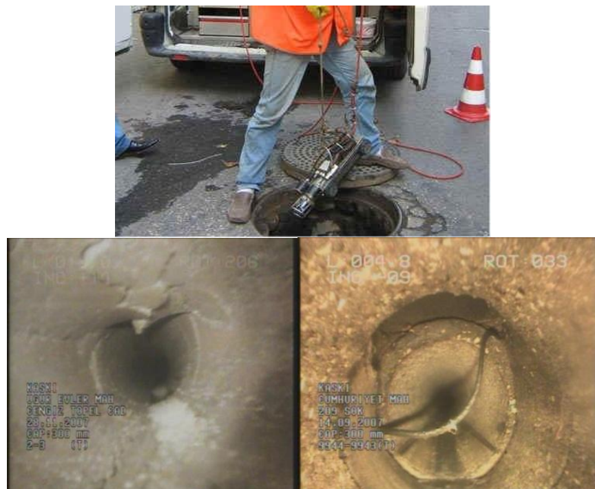
Figure 2.6. Obtaining image of the water distribution system while cleaning via image endorser robot (Nalbantoğlu, 2010).
