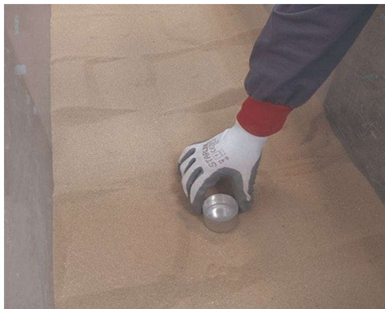
Figure 3.12. Placement of Density Cans on the Backfill.
