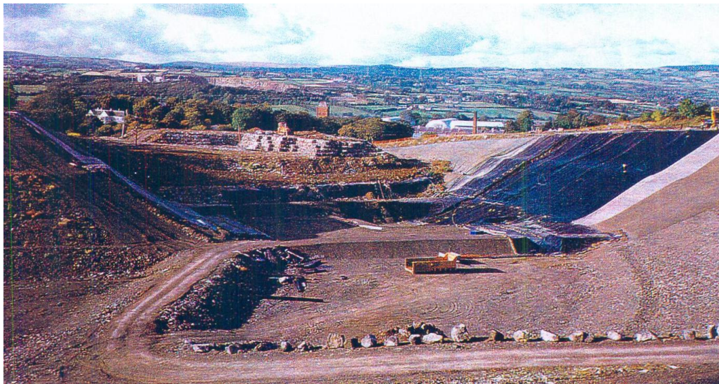
Figure 2.5 Geomembrane and Geotextile applications
