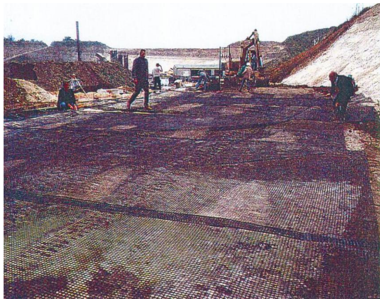
Figure 2.4 Geogrid reinforced pavement construction
