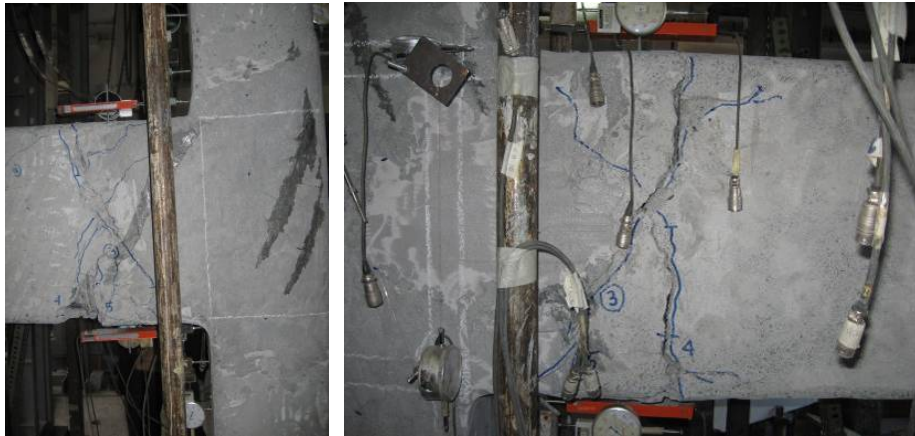
Figure 3.6. Final crack patterns of beam
