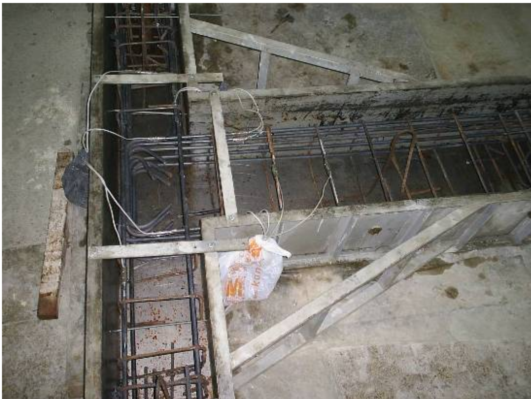
Figure 2.28. A Picture from Construction of Specimen TR-5 Control
