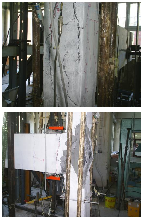
Figure 3.17. Cracking of joint region at the end of the test
