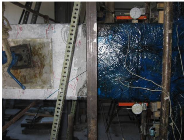
Figure 3.11. Cracks formed on the beam
