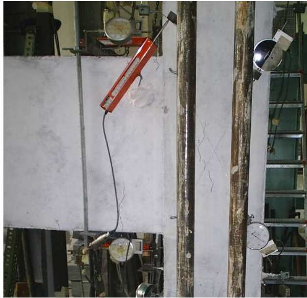
Figure 3.19. The first shear crack in the joint
