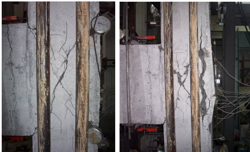
Figure 3.3. Crack pattern at 2.20% and 2.75% drift level
