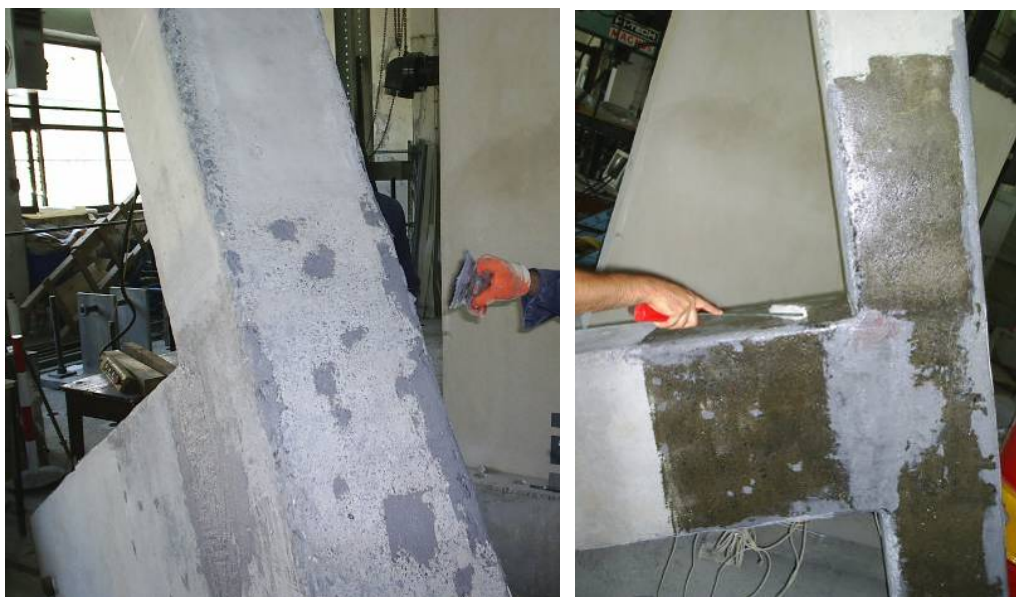
Figure 2.16. Surface preparation and application of MBrace Primer.
