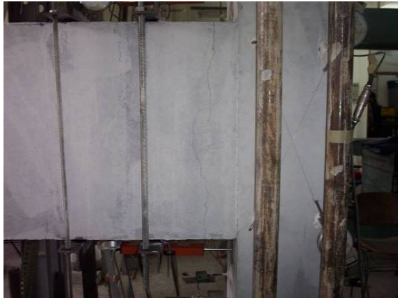
Figure 3.14. Flexural cracks up to the drift level of 0.35%
