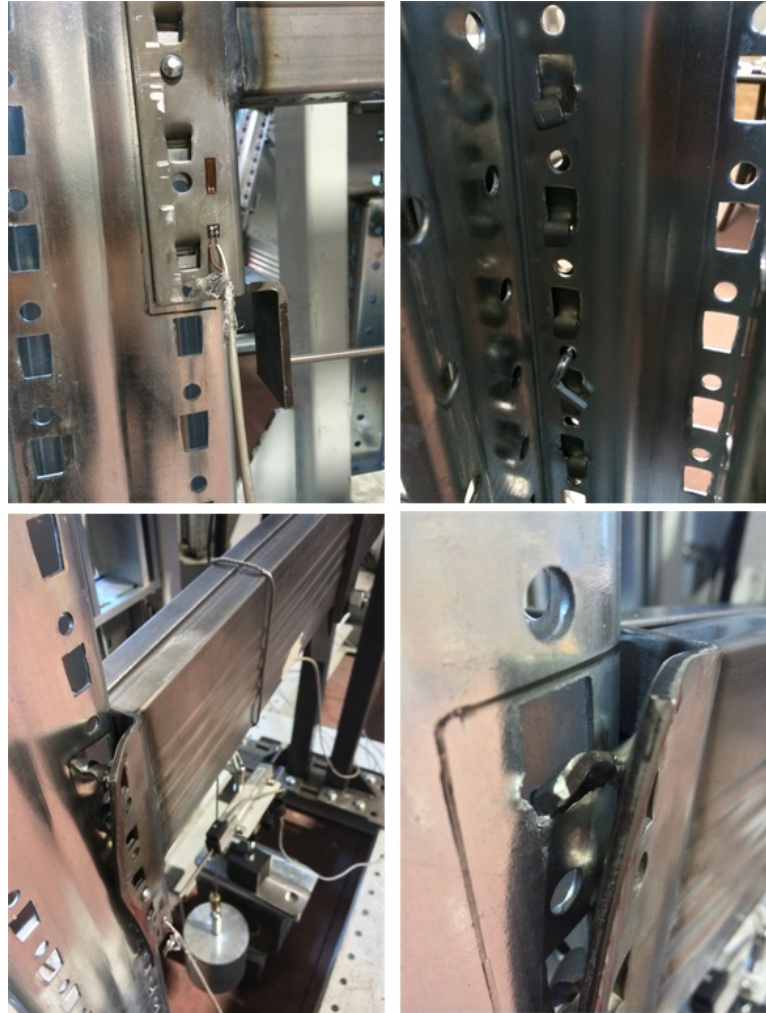
Figure 3.41. Collapse Modes in TC150.
