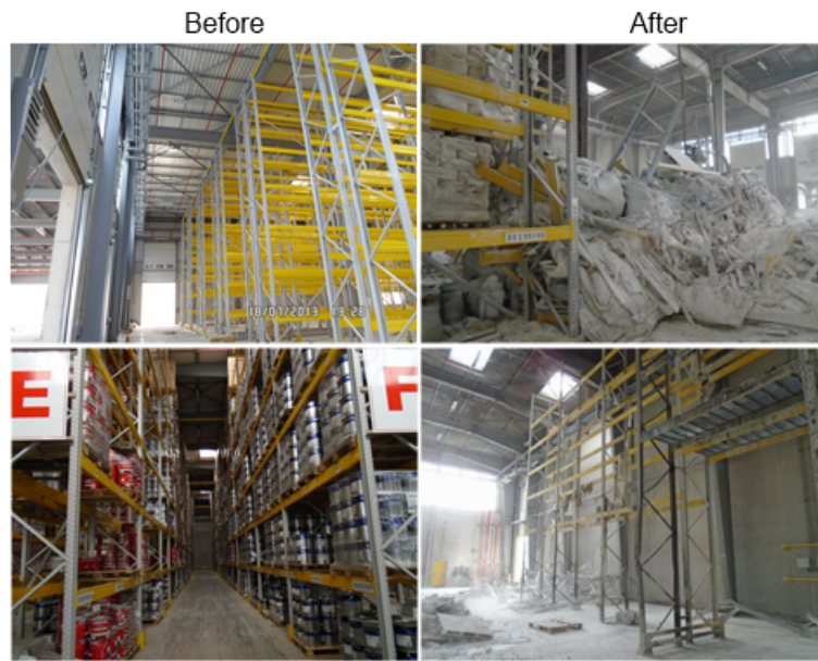
Figure 1.5. Rack Collapse Due to Incorrect Design.
