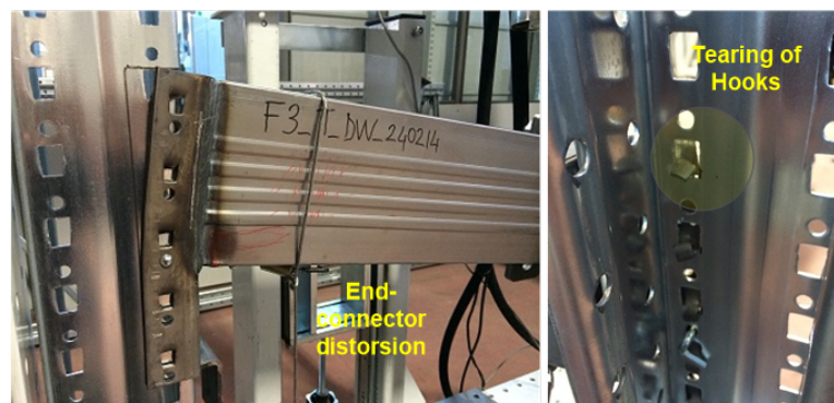
Figure 3.20. Failure Modes in Monotonic Tests on TP140 Specimens - Back Face.
