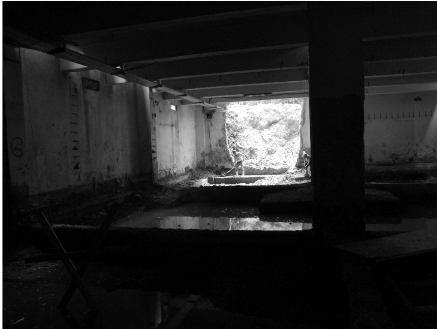
Figure 3.5. Foundation During Retrofitting.
