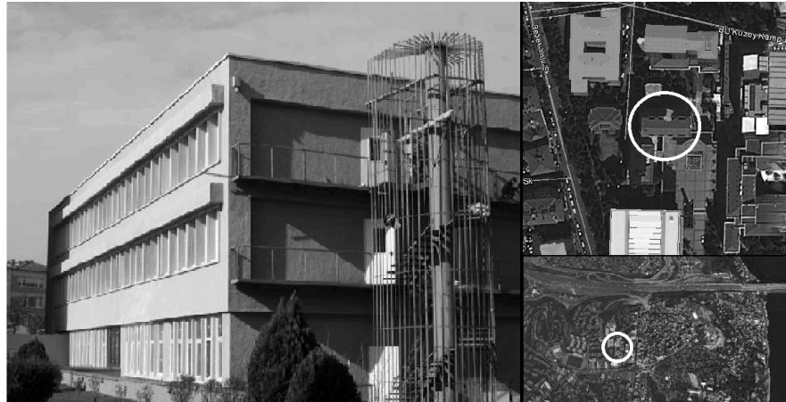
Figure 3.4. ETA-B Building and Its Location.
