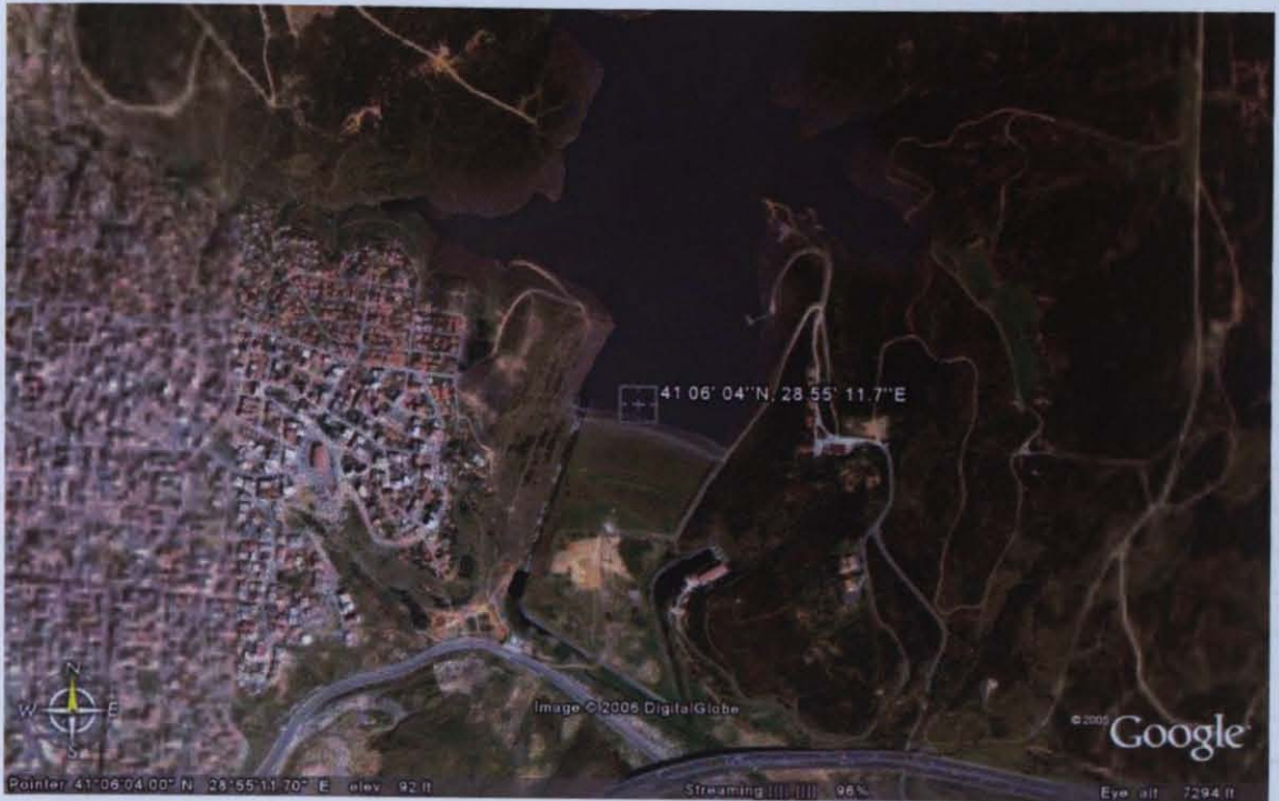
Figure 2 - 3: Satellite view of Alibey Earth Dam. Courtesy of Google Incorporation. Google Earth Virtual Globe Software, 2006.
