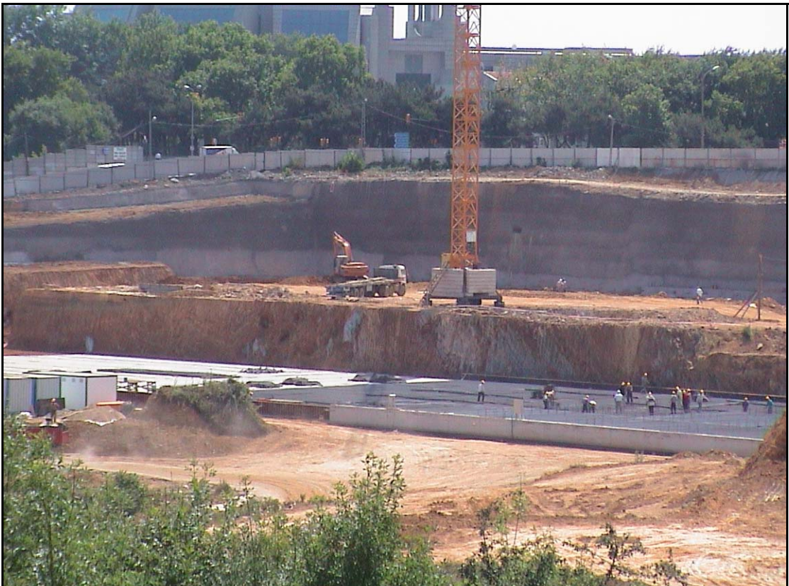
Figure 5.17. A photograph from Istinye Park Complex, inclinometer 4 section
