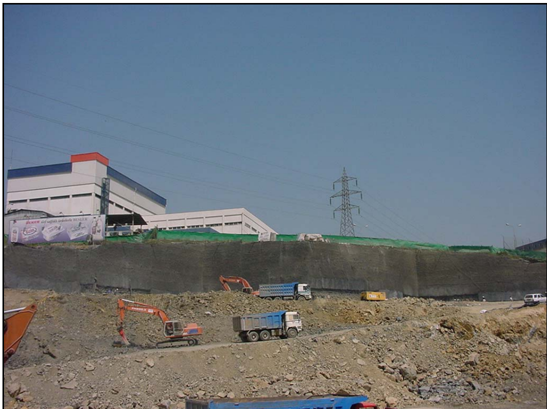
Figure 5.29. A photograph from Besler Warehouse, inclinometer 1 section
