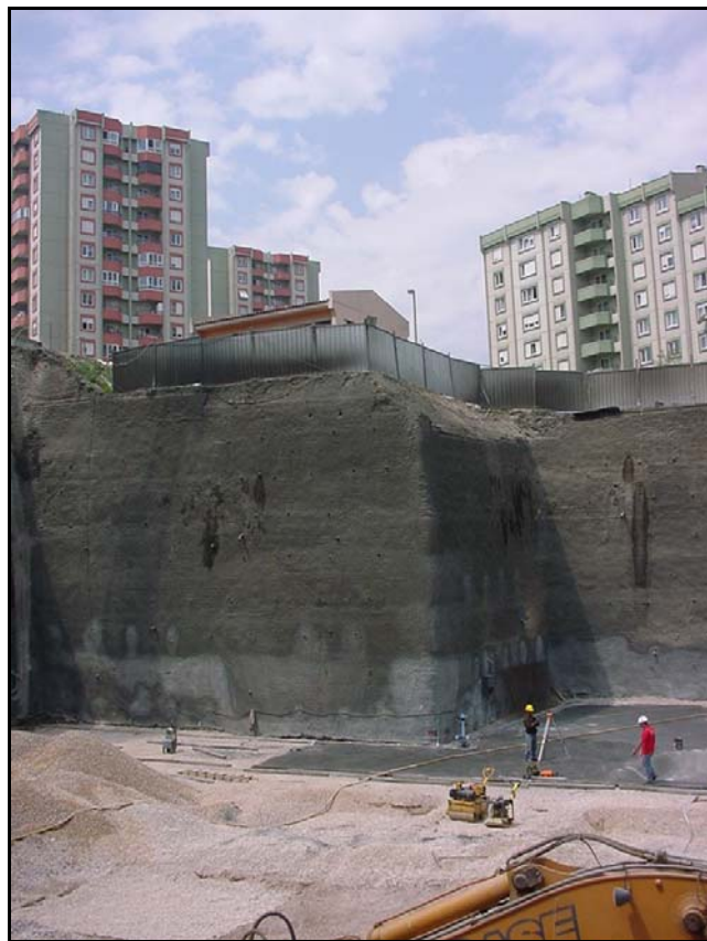
Figure 3.14. Separate soil nailing application for a deep excavation in Istanbul (Zetas, 2006)
