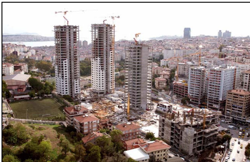
Figure 7.4. BJK Fulya Complex, during the construction, September 2007
