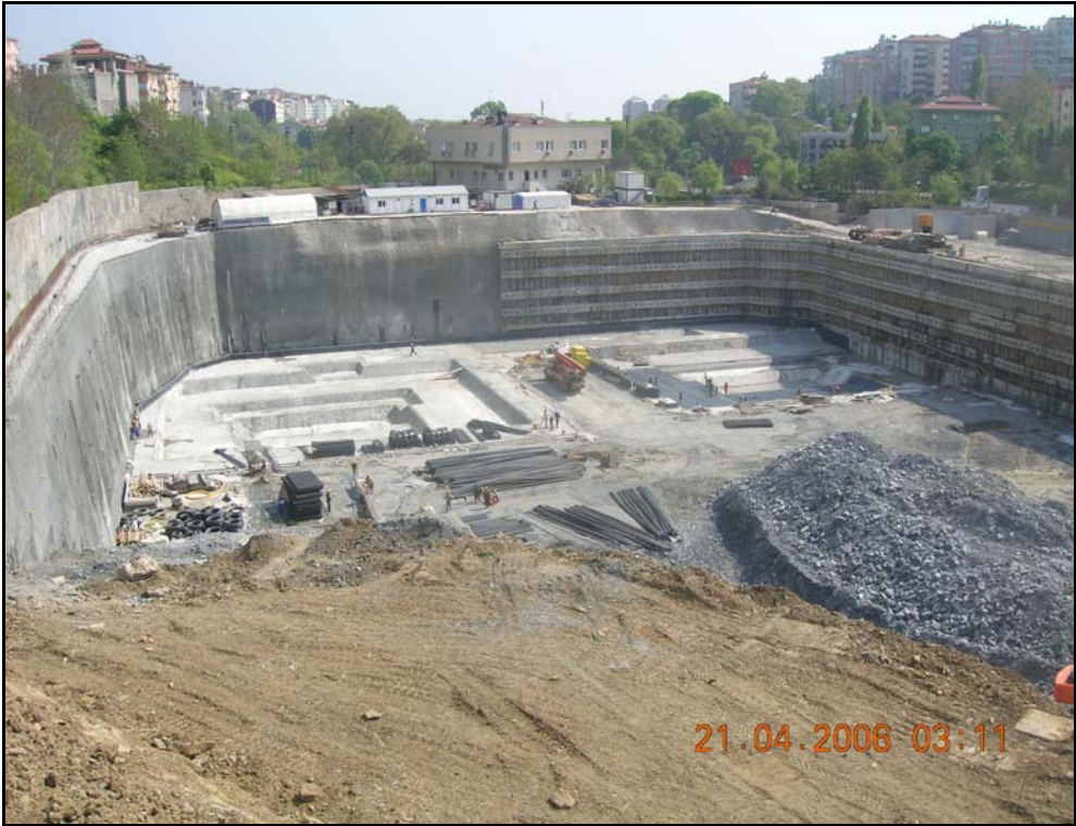
Figure 7.24. Retaining system facing north side
