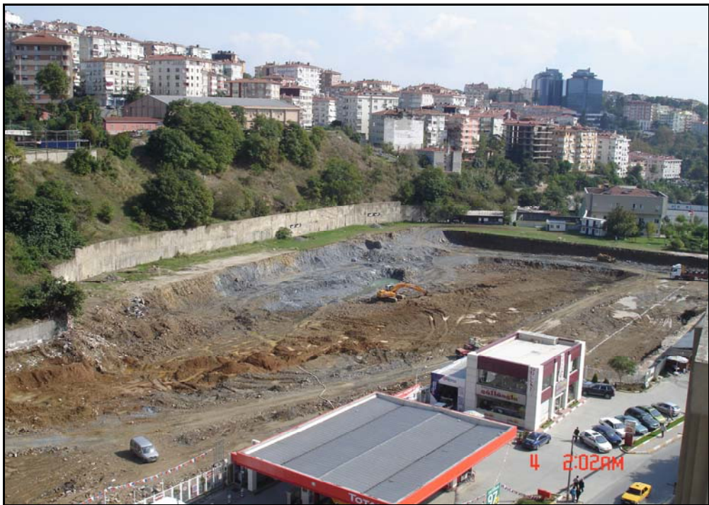
Figure 7.6. A picture from early stages of excavation, September 2005
