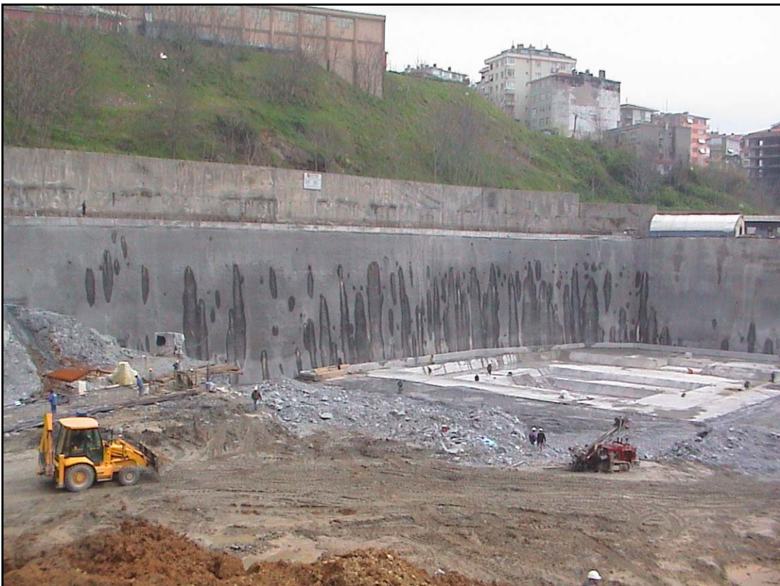
Figure 5.14. A photograph from BJK Fulya Complex, inclinometer 1 section
