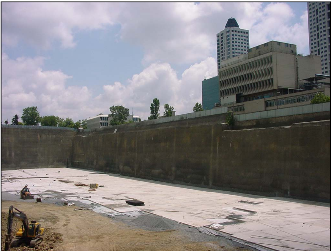
Figure 5.20. A photograph from Kanyon Complex, inclinometer 7 section
