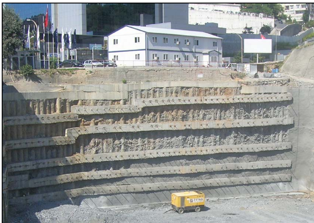
Figure 7.23. Cast in-situ reinforced concrete walls in segments under the bored piles
