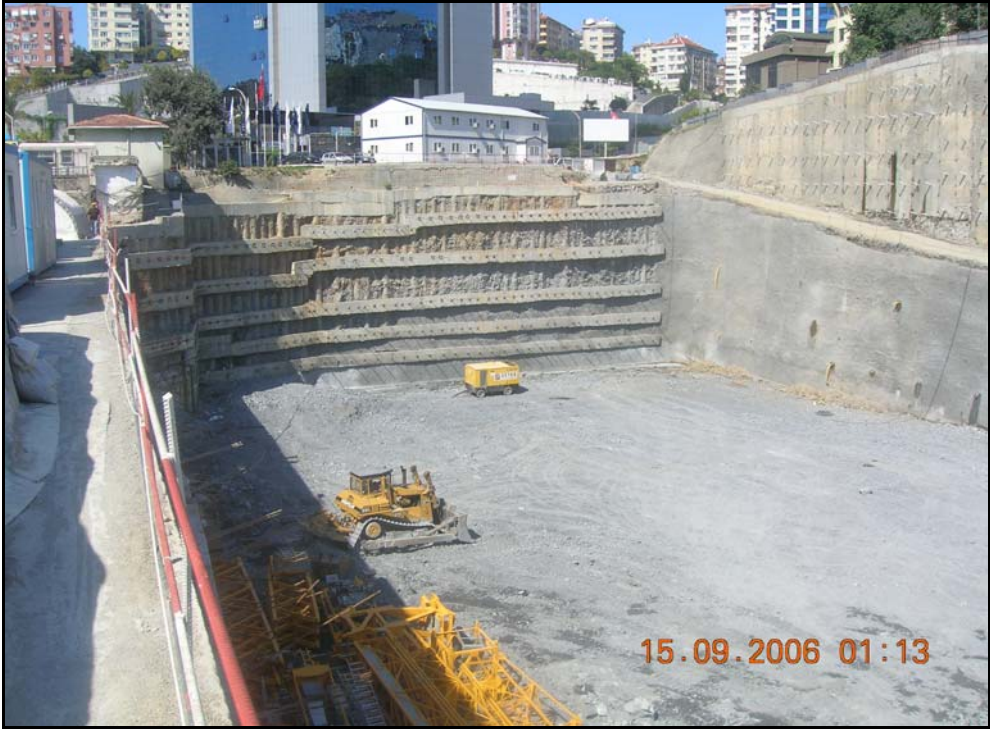
Figure 7.25. Retaining system facing south side
