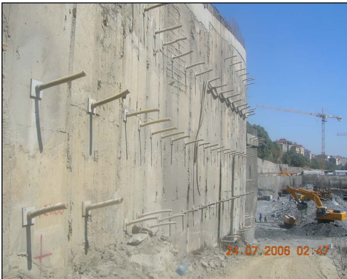
Figure 7.9. A picture from caisson wall of Type 1
