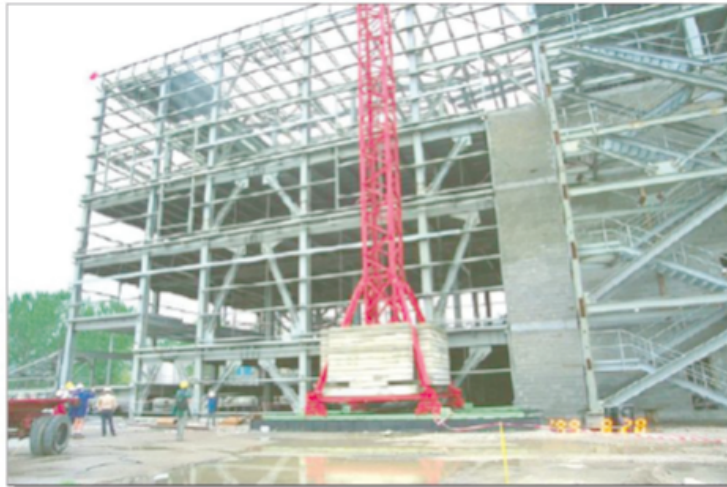
Figure 5.2. Example of EBF Application (SEAOC 2000).
