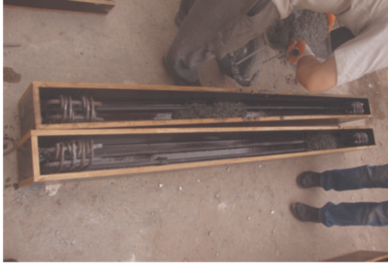
Figure 3.1. Image of beam reinforcement.
