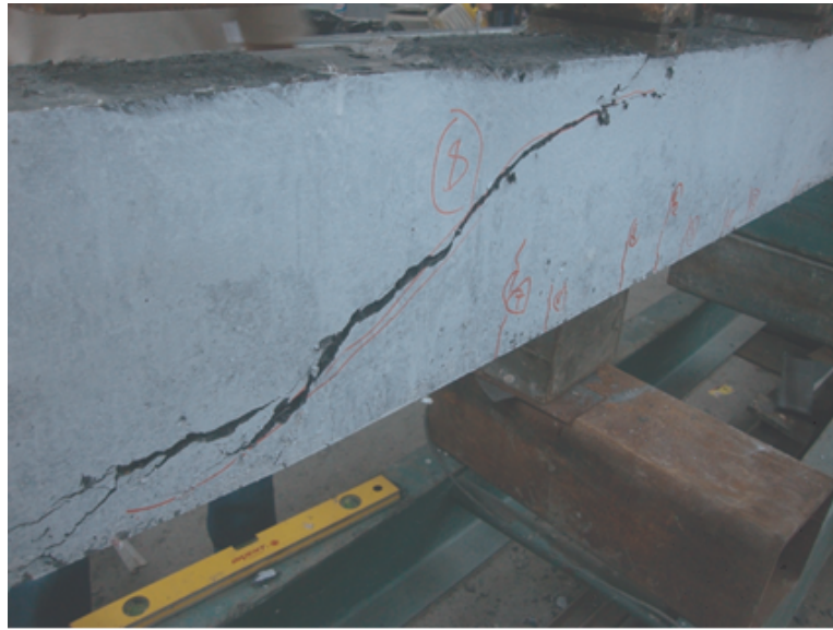
Figure 4.23. Crack propagation and damaged shape of B-08.
