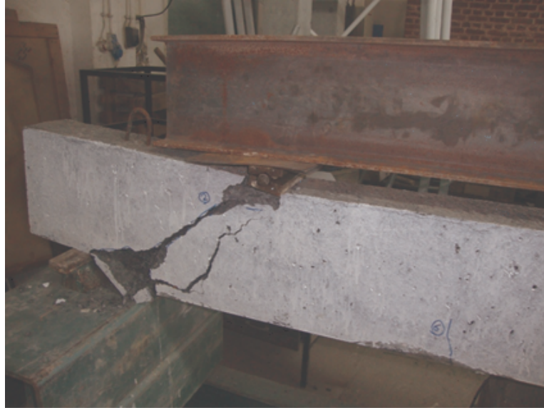
Figure 4.4. Damaged shape of B-01.
