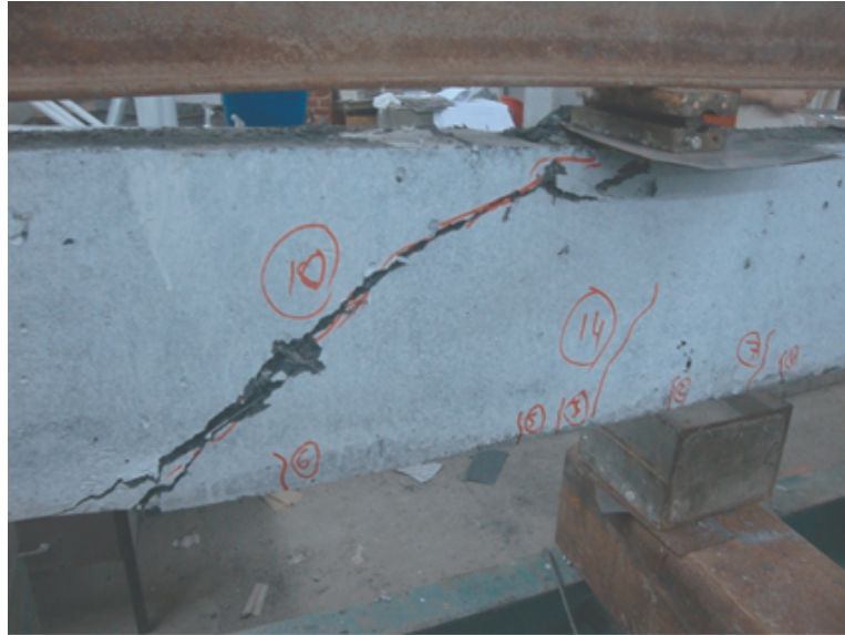
Figure 4.29. Damaged shape of B-10.
