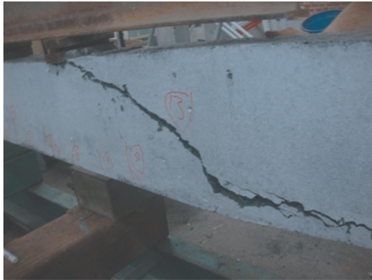
Figure 4.18. Damaged shape of B-06.
