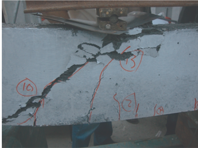
Figure 4.21. Damaged shape of B-07.
