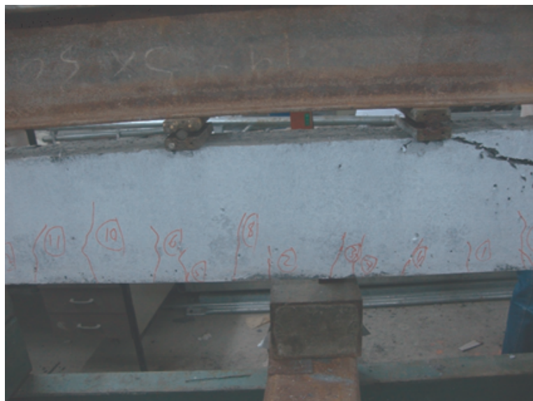
Figure 4.17. Crack propagation of B-06.
