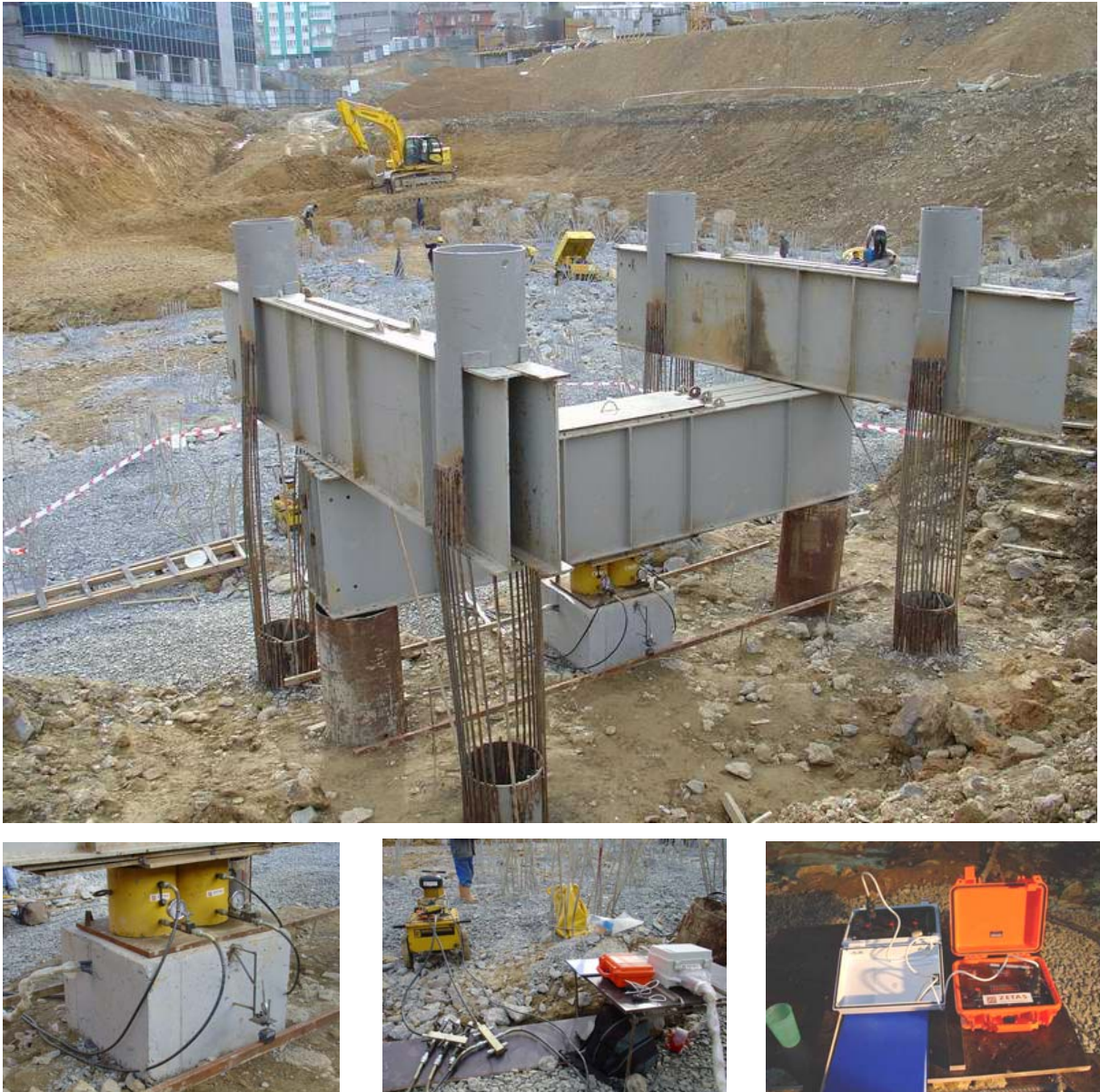
Figure 4.13. Test pile reaction system site pictures
