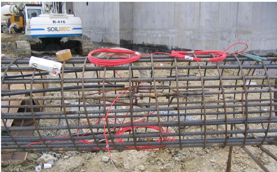
Figure 4.5. Installation of vibrating wire strain gauge on piles
