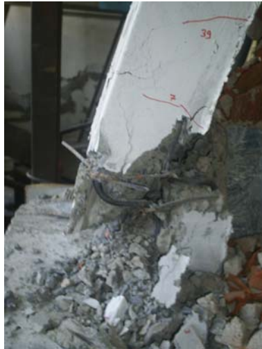
Figure 4.54. Close-up of left column at the end of the test
