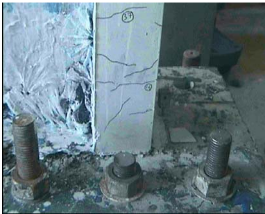
Figure 4.31. Close-up of the right column
