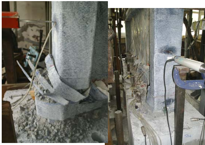
Figure 4.72. Close-up of the left and right columns after the test
