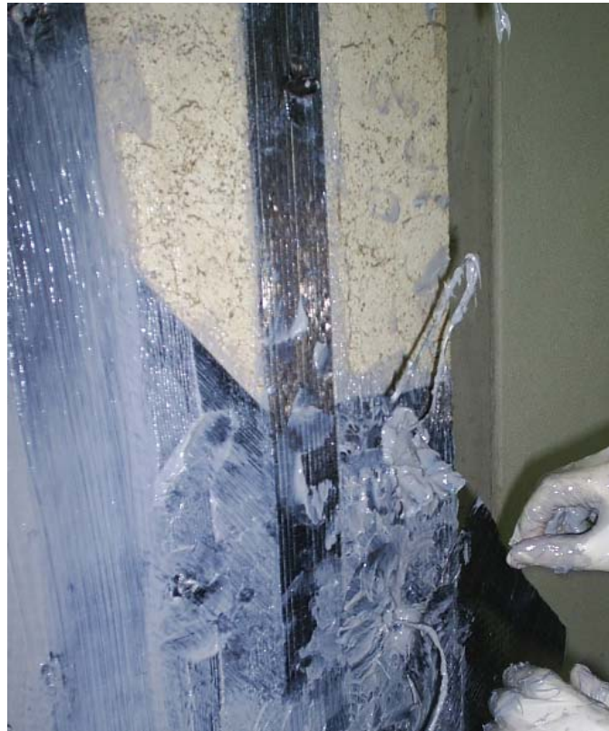
Figure 3.14. Placement of anchors
