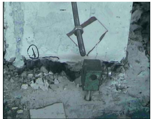
Figure 4.32. Close-up of the left column
