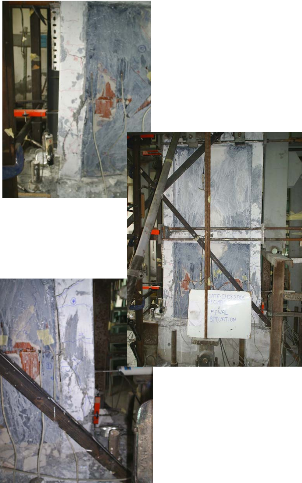
Figure 4.18. Specimen SA1.0-C2V at the end of the test
