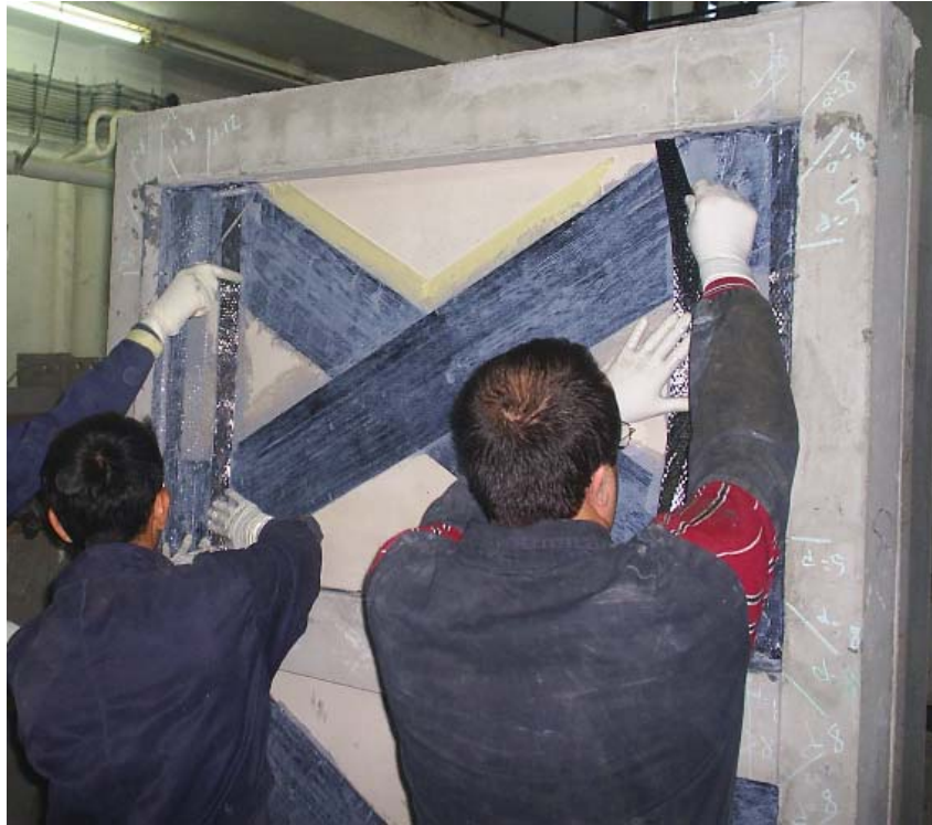
Figure 3.13. Application of vertical strips
