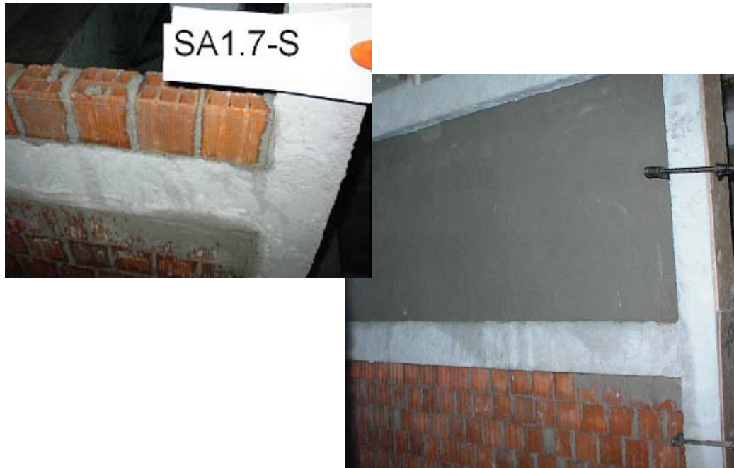
Figure 3.9. Laying of bricks and plastering of the brick wall
