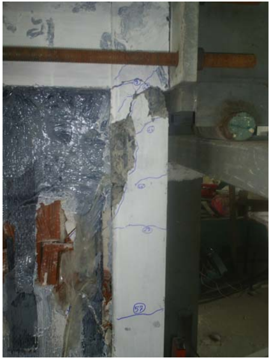
Figure 4.42. Close-up of the right column top end
