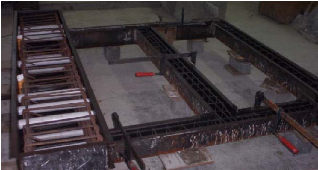
Figure 3.8. Picture of reinforcement cage prior to casting of concrete.
