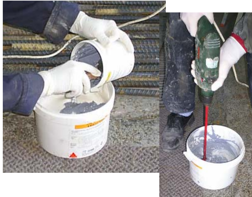
Figure 3.11. Preparation of the epoxy resin
