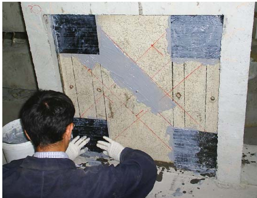
Figure 3.12. Application of corner flags
