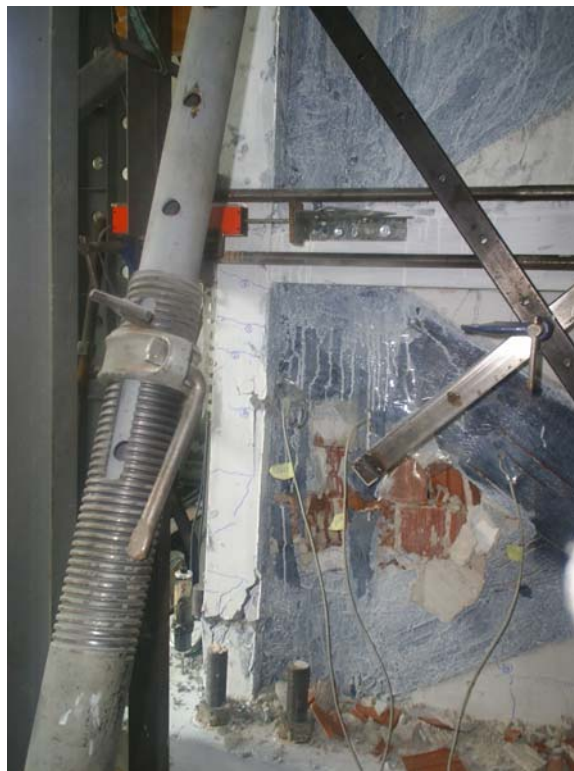
Figure 4.40. Close-up of the left column
