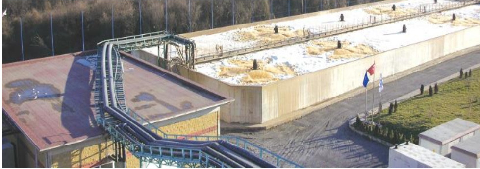
Figure 7.7. Kemberburgaz Leachate Treatment Plant
