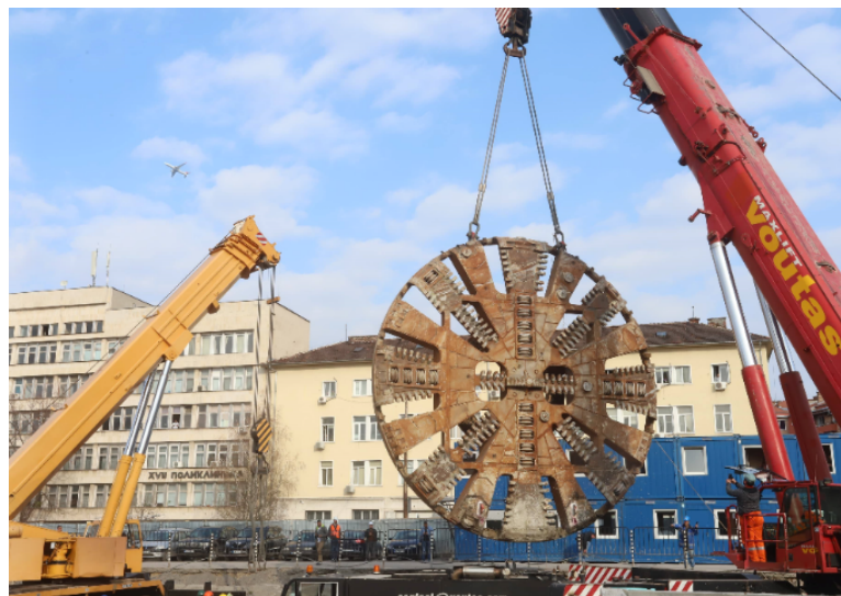
Figure 5.12. Cutterhead during TBM Disassembly.
