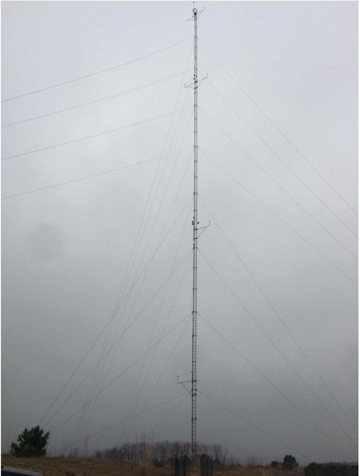
Figure 3.5. The weather station near the wind turbine
