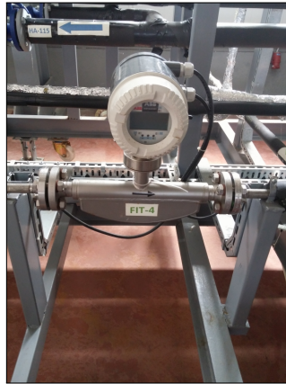
(b) Coriolis flowmeter
