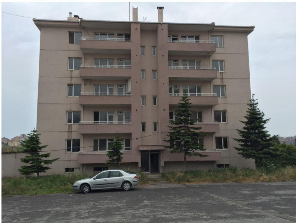
Figure 2.1. Front view of the building.
