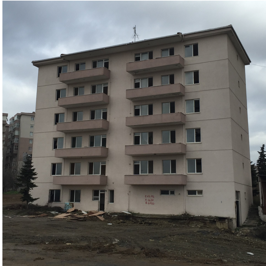
Figure 2.2. Rear view of the building.
